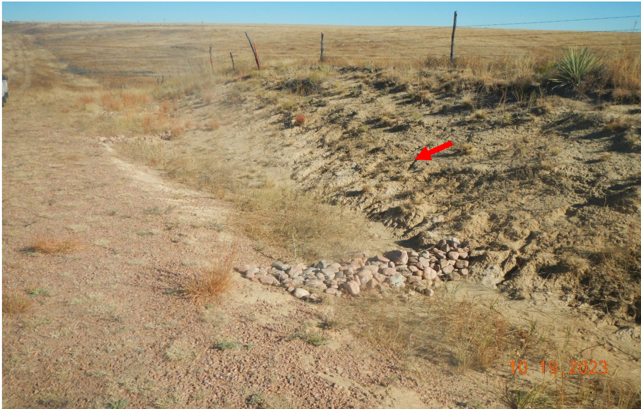
Photo 4. Facing northeast along the road toward the erosion along the roadside. There has been additional rock check dams installed however there is erosion at red arrow that needs to be stabilized and seeded.
