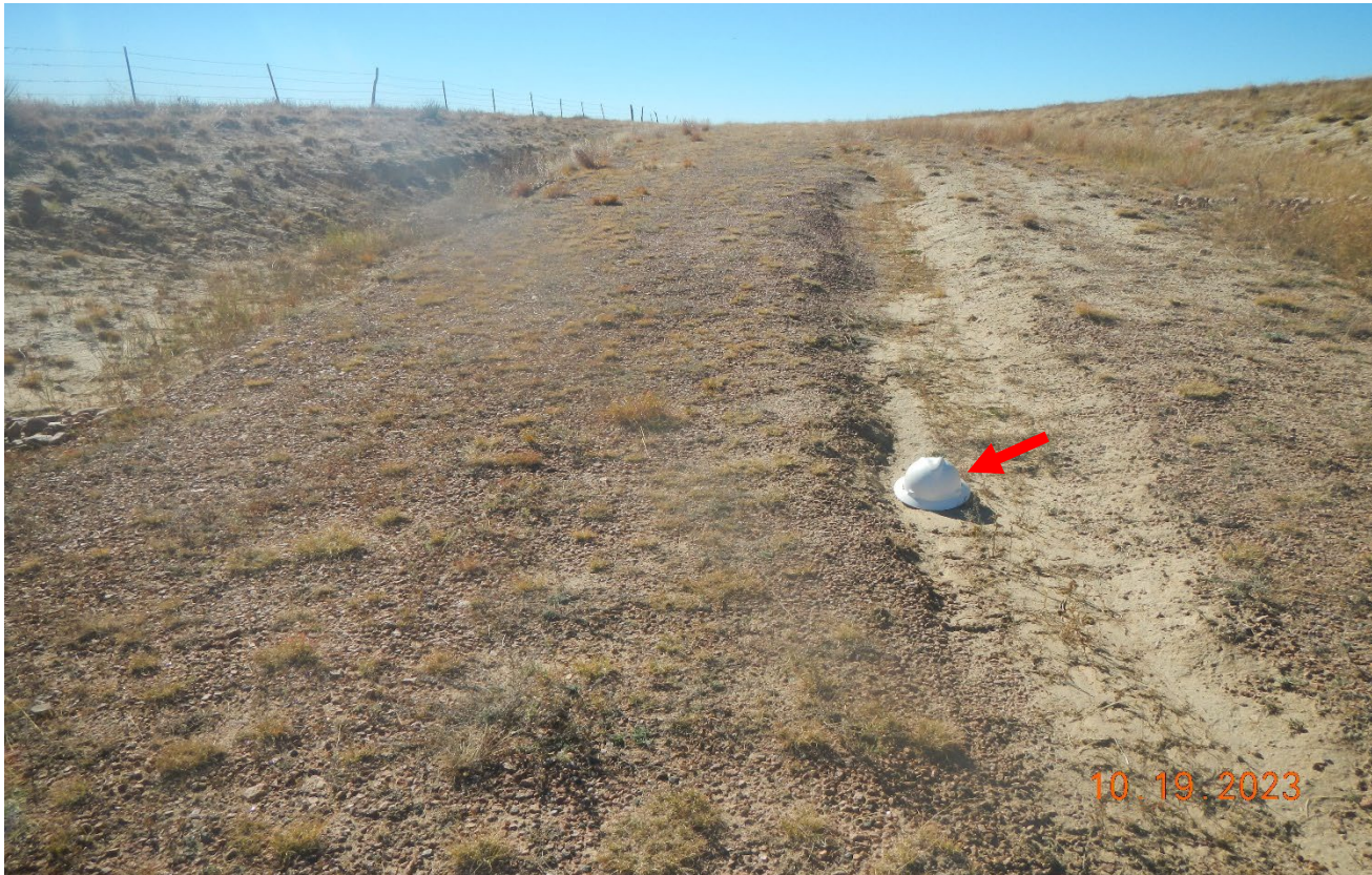
Photo 2. There is an erosion channel along the road at LatLong:38.74925,-104.55225. This area needs to be repaired and stabilized. Red arrow points to hard hat in the erosion channel.
