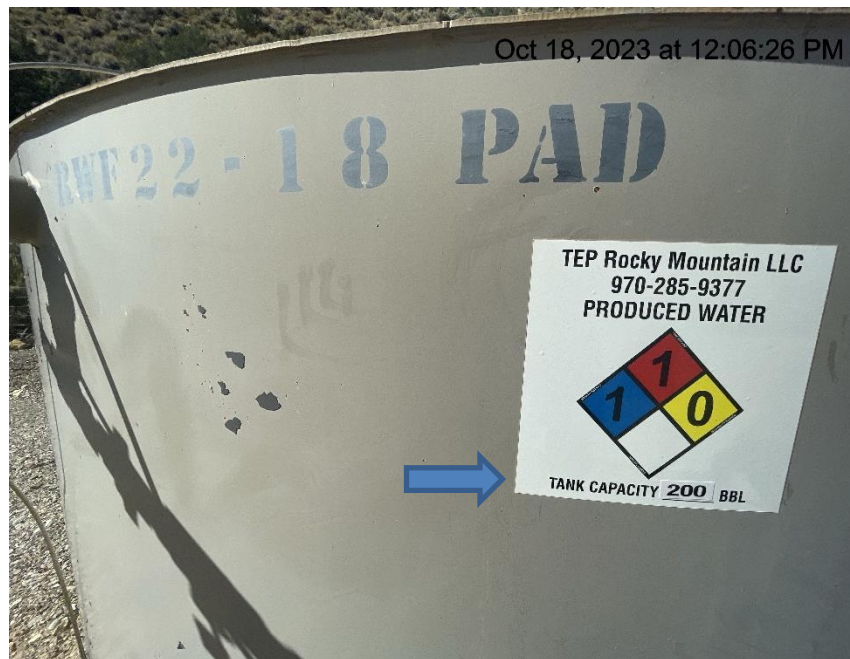
Photo # 2924 Tank label has incorrect capacity
