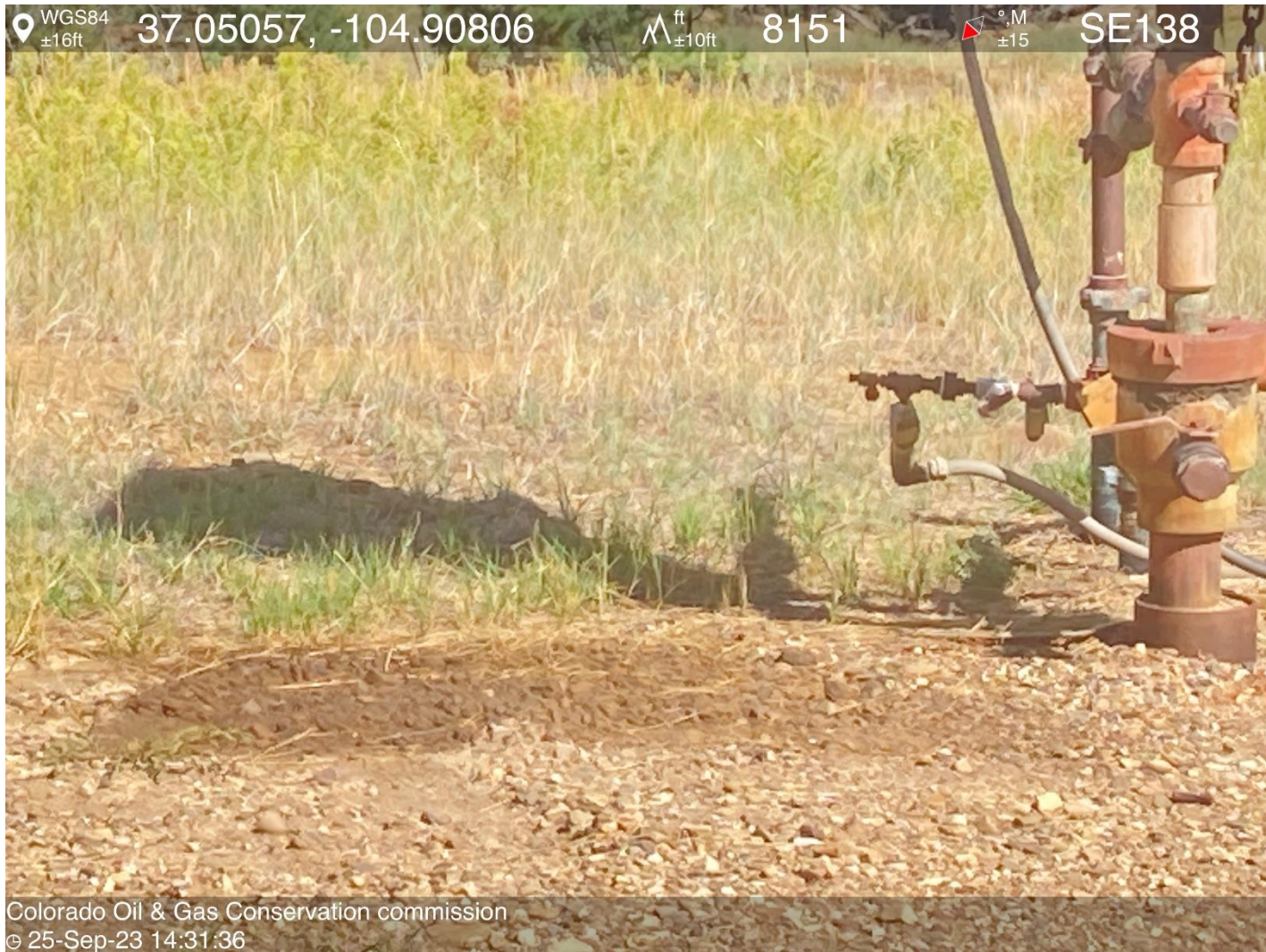
PHOTO 5: AREA OF IMPACTED SOIL APPEARS TO BE FROM A PREVIOUS HYDRAULIC HOSE LEAK (NO LEAK AT TIME OF INSPECTION). Conduct maintenance on equipment, cleanup stained material and review self inspection processes. COMPLY WITH RULE 1002,(2).D. CA DATE 11-19-2023.
