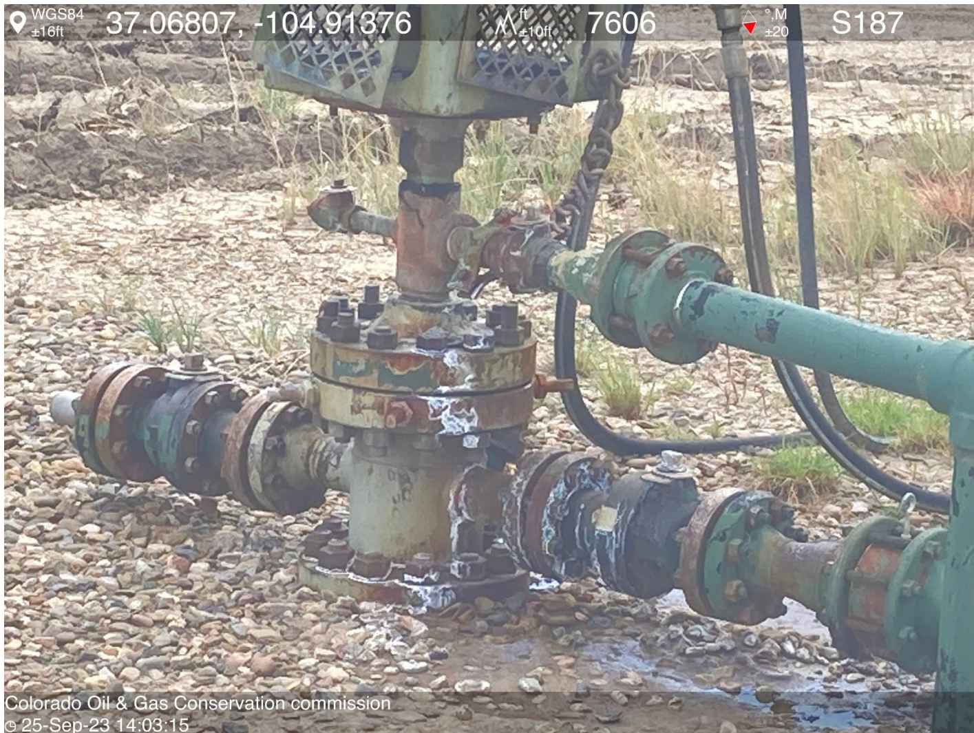
PHOTO 5: Signs of recent slow leak from wellhead. Salt/mineral buildup is evident on the wellhead. Securely fasten all valves, pipes, fittings, and Production Facilities to ensure good mechanical condition, remove salt/mineral buildup, inspect at regular intervals and maintain in good mechanical condition per Rule 608.e. CA DATE 11-19-2023.
