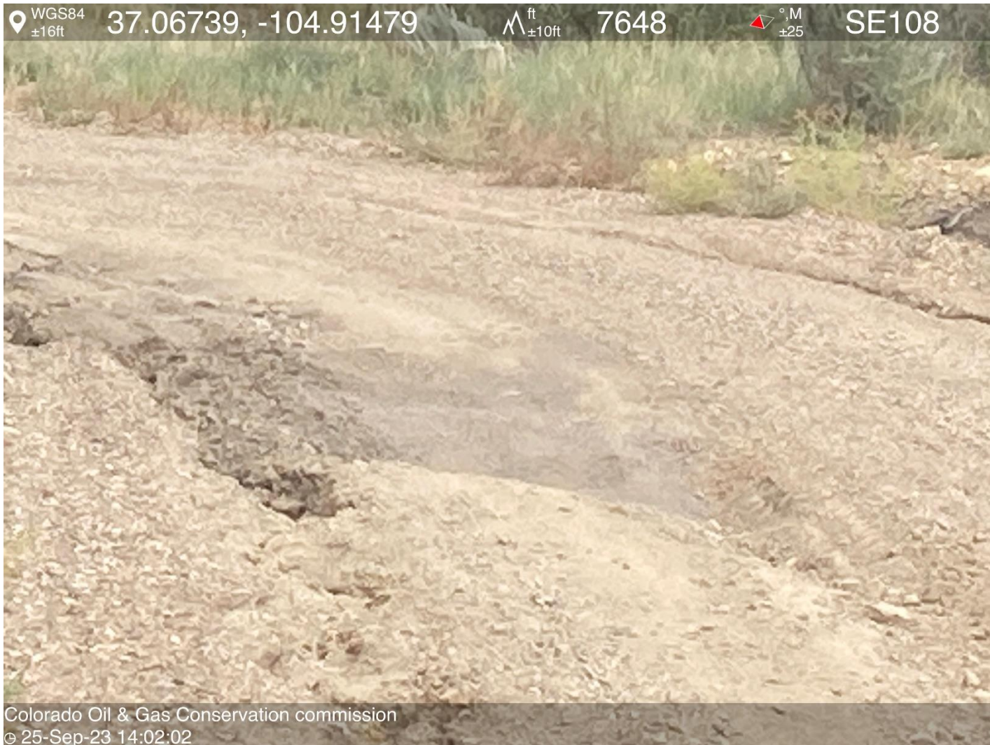
PHOTO 9: NO STORM WATER BMP'S INSTALLED OR BMP'S ON ROW DRAINAGE DITCH JUST SOUTH OF LOCATION HAS CAUSED EROSION ON AND ALONG SIDE ROW. Install or repair required BMPs per Rule 1002.f.(2)C CA DATE 11-19-2023.
