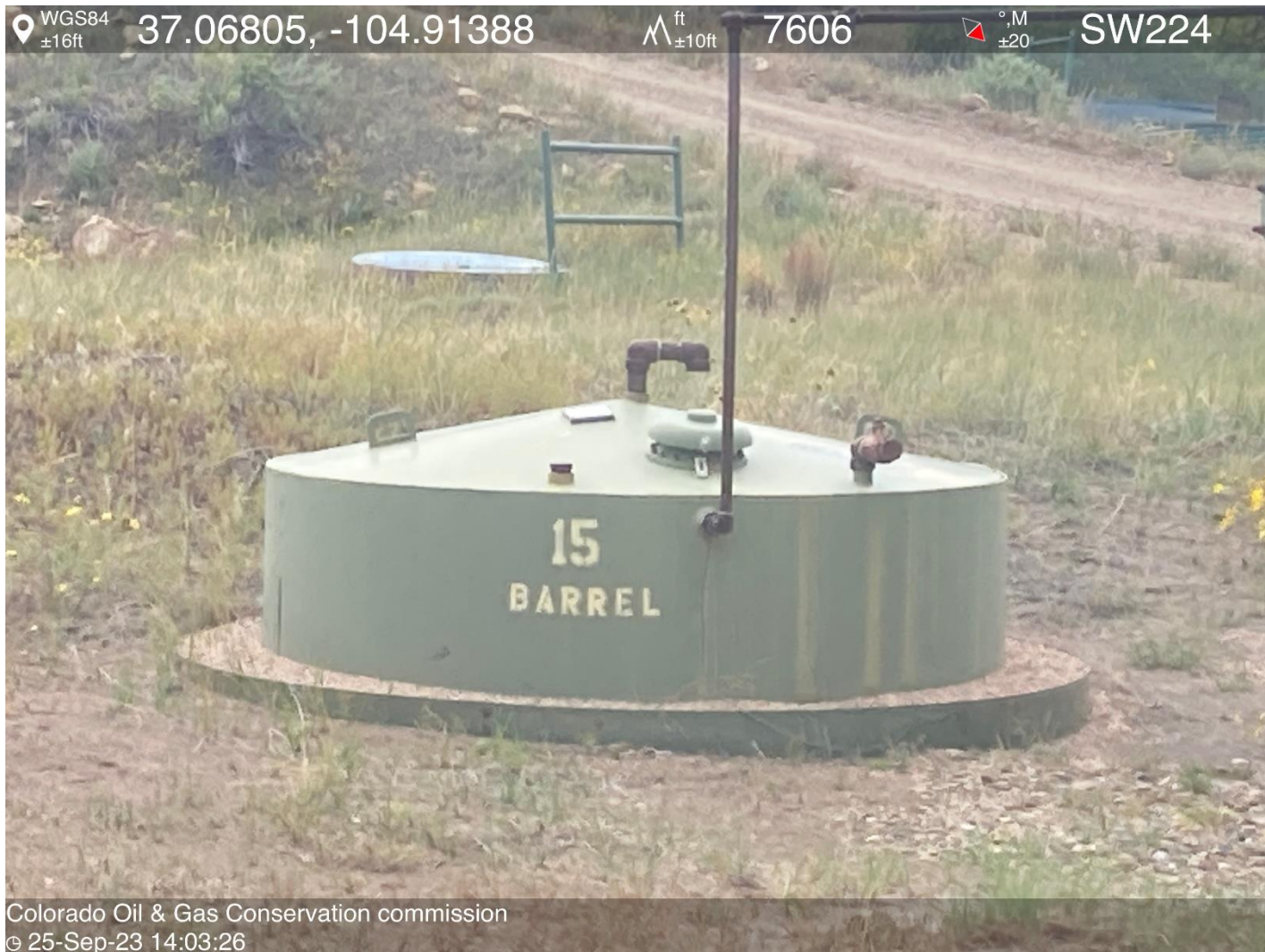
PHOTO 4: 15 BBL PRODUCED WATER TANK.
