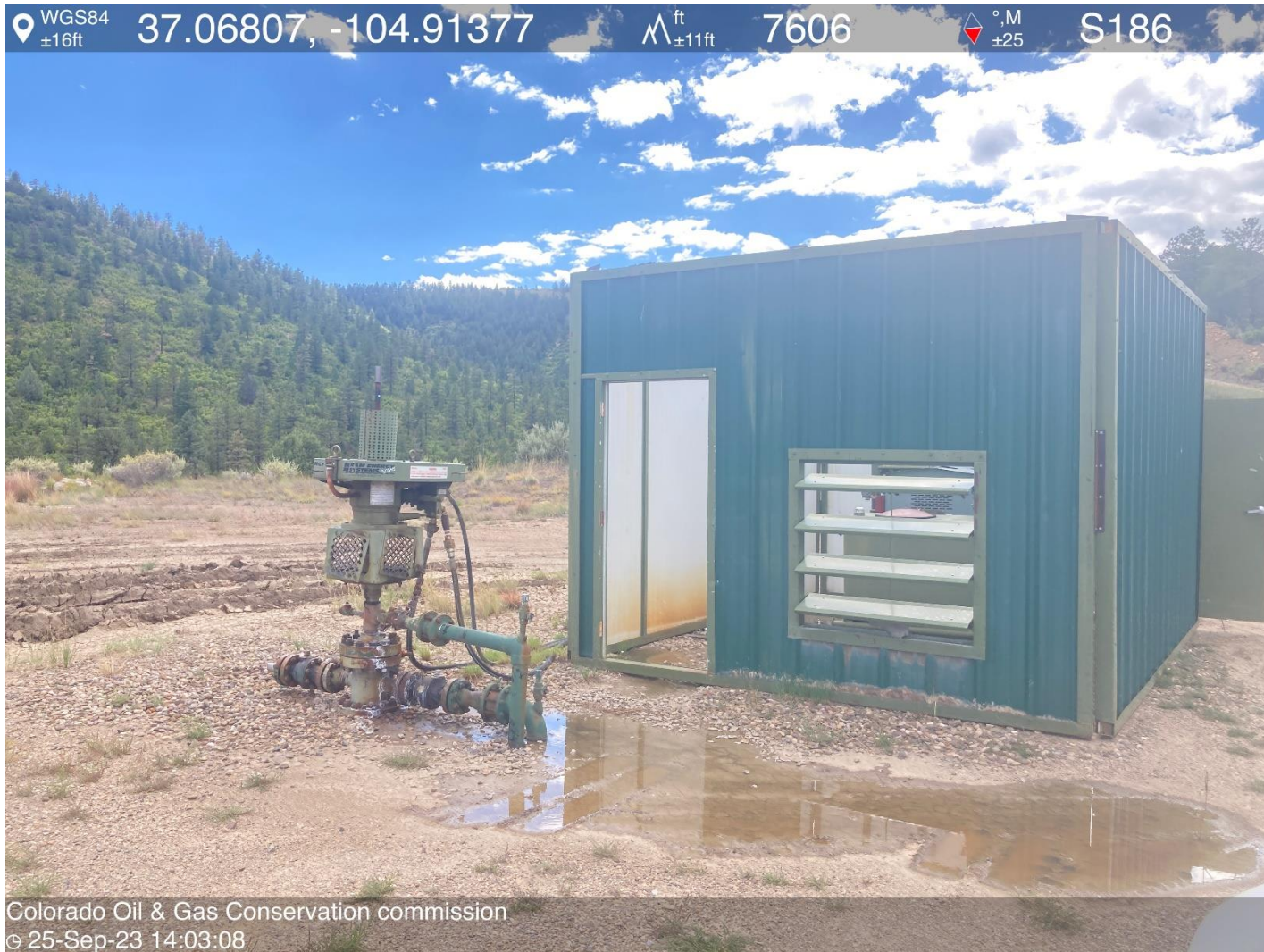
PHOTO 6: Produced water spill from the wellhead has left a salt impacted area around the wellhead. Securely fasten all valves, pipes, fittings, and Production Facilities to ensure good mechanical condition, inspect at regular intervals, remove salts/mineral impacted soils, and maintain in good mechanical condition per Rule 608.e. CA DATE 11-19-2023.
