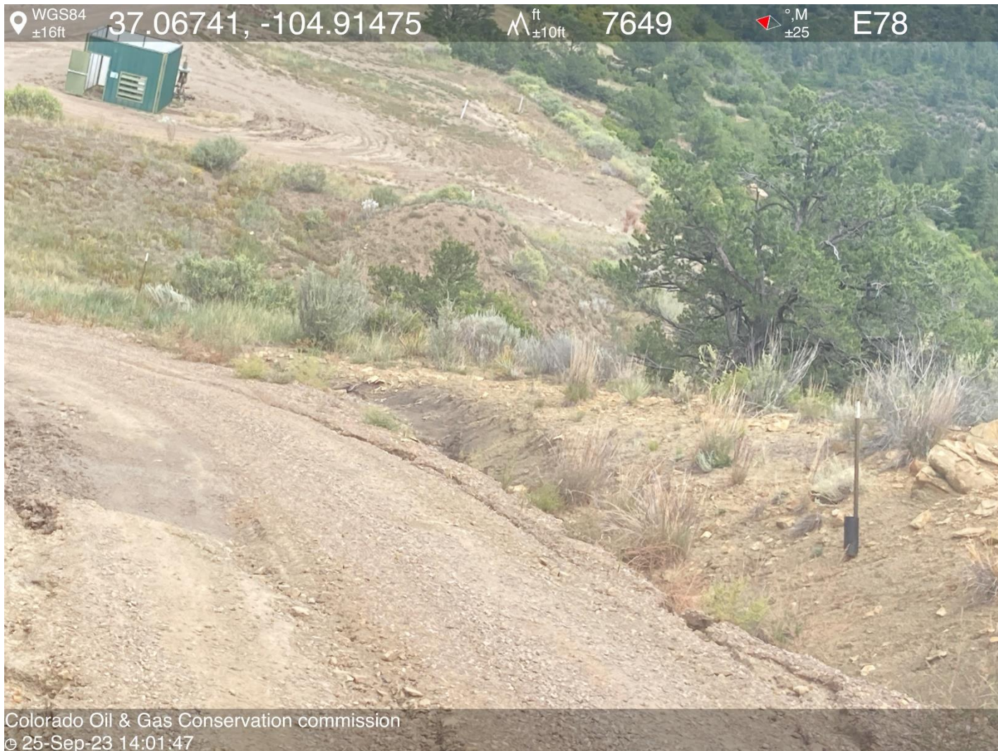
PHOTO 8: NO STORM WATER BMP'S INSTALLED OR BMP'S ON ROW DRAINAGE DITCH JUST SOUTH OF LOCATION HAS CAUSED EROSION ON AND ALONG SIDE ROW. Install or repair required BMPs per Rule 1002.f.(2)C CA DATE 11-19-2023.
