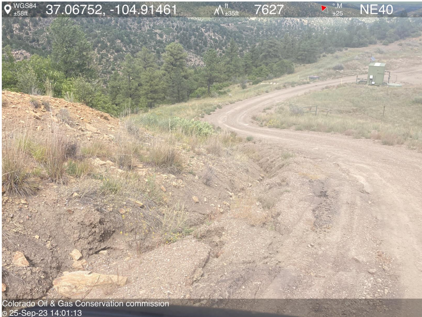
PHOTO 7: NO STORM WATER BMP'S INSTALLED OR BMP'S ON ROW DRAINAGE DITCH JUST SOUTH OF LOCATION HAS CAUSED EROSION ON AND ALONG SIDE ROW. Install or repair required BMPs per Rule 1002.f.(2)C CA DATE 11-19-2023.
