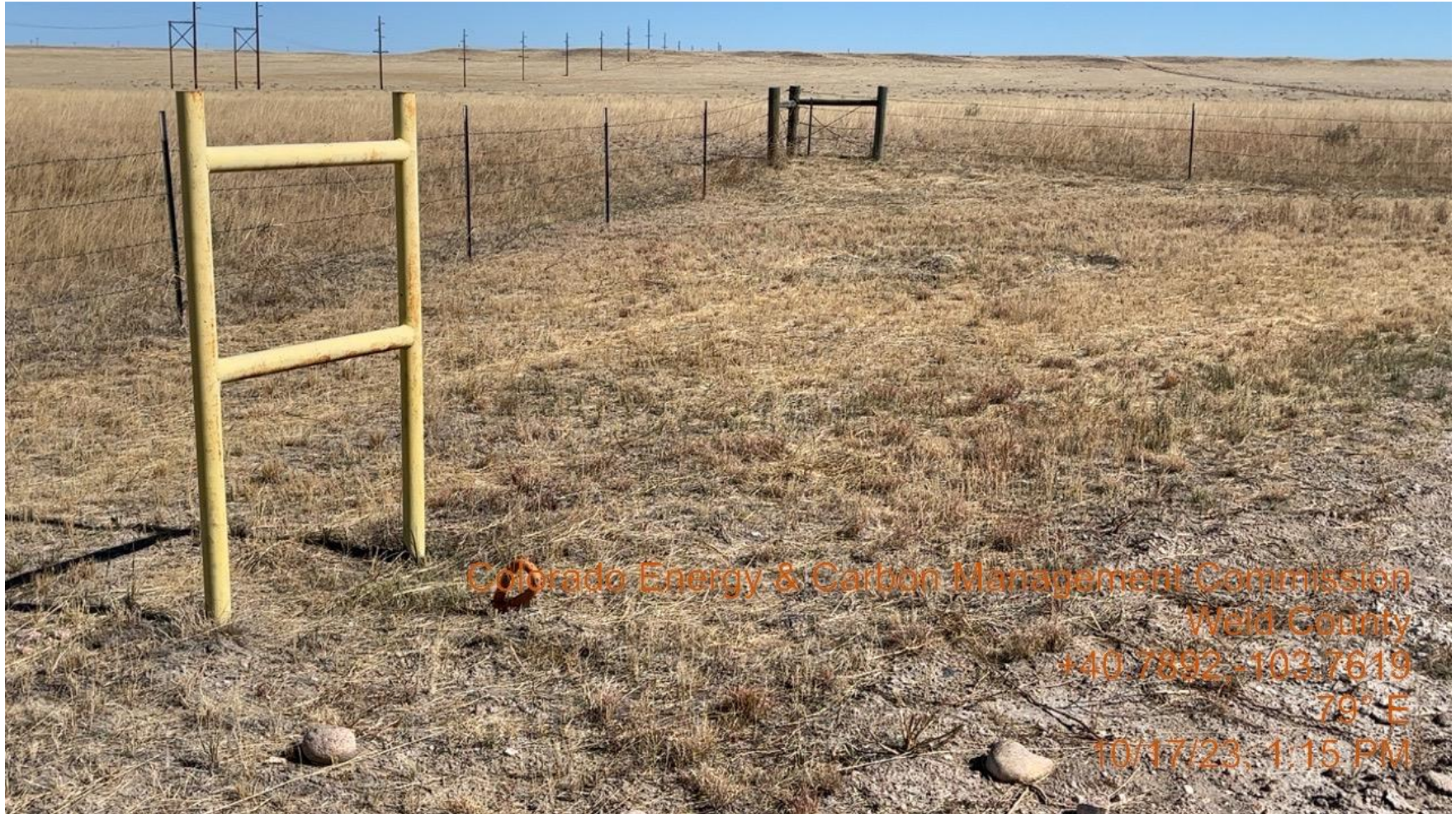
Photo 3. Photo on location facing East. The photo illustrates the guy line anchors are visibly marked by yellow painted steel uprights. The photo also illustrates there has been good recruitment of vegetation in the interim but that it has been mowed.
