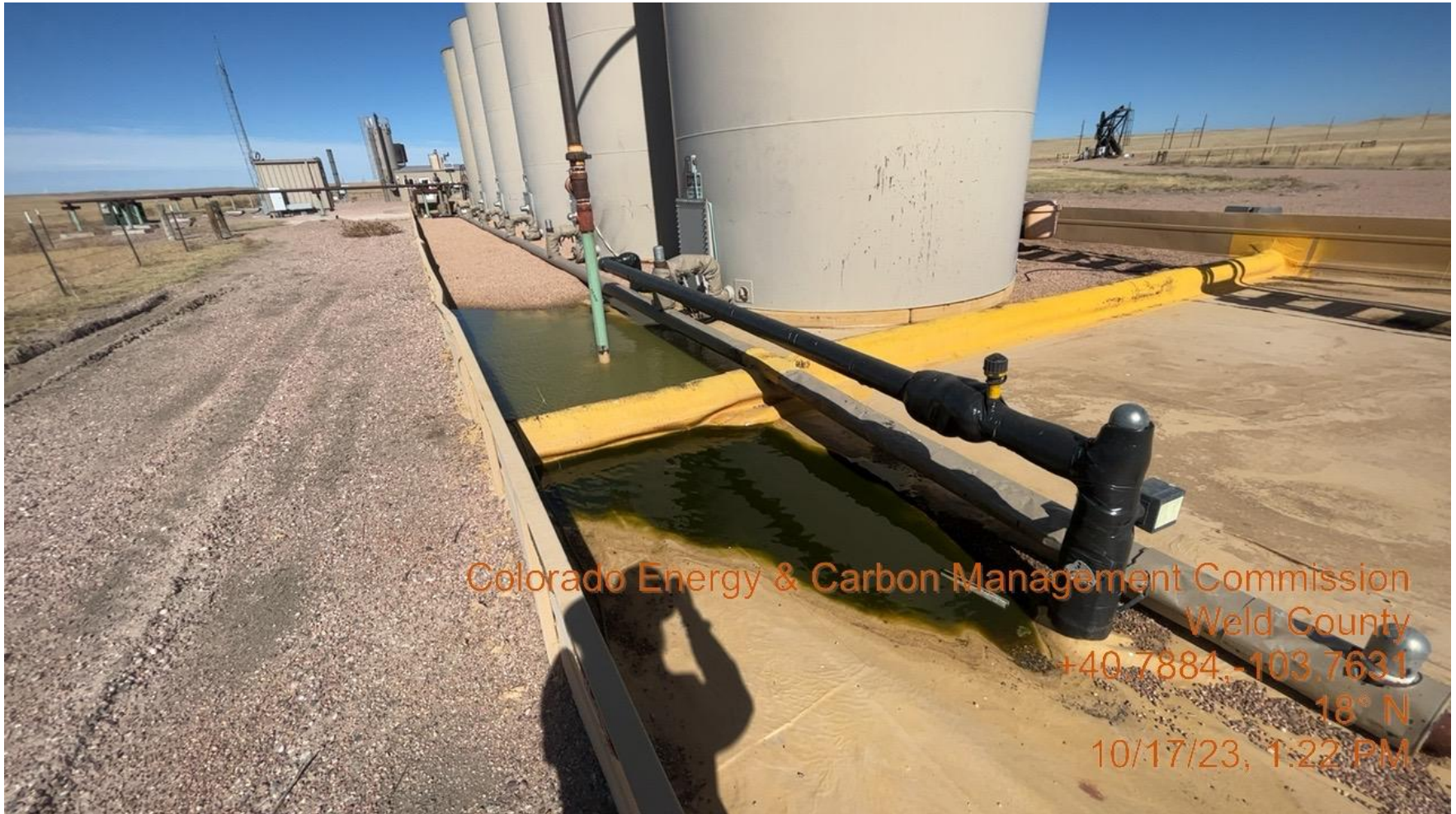
Photo 5. The photo was taken from the West side of the location facing North. The photo illustrates produced water inside the secondary containment.
