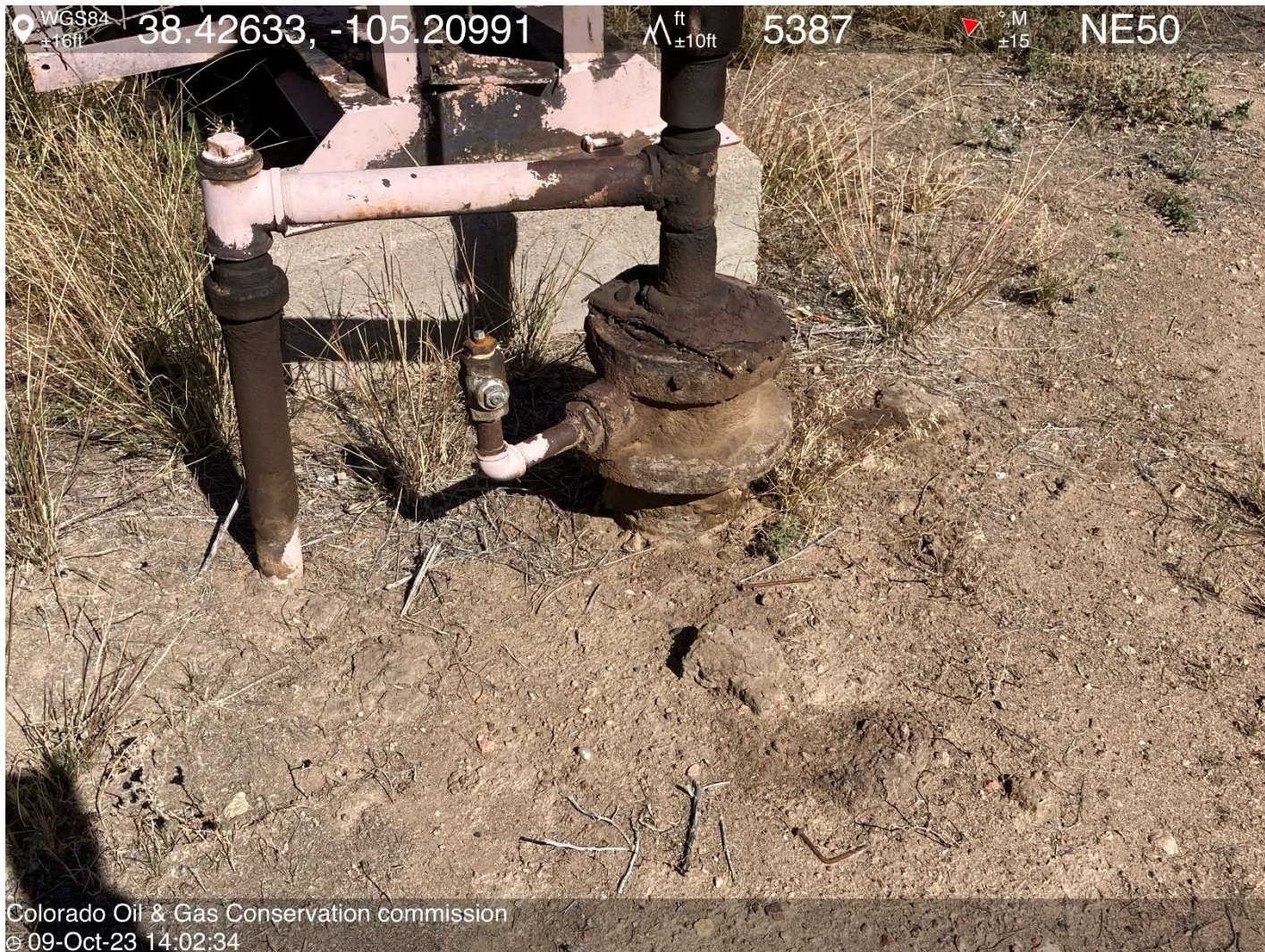
PHOTO 12: BRADENHEAD IS NOT ACCESSABLE. Install appropriate fittings to allow bradenhead visual inspection as per Rule 419.a.(1), (2). CA DATE 11-19-2023.
