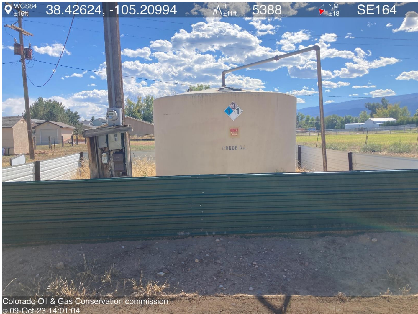
PHOTO 4: TANK BATTERY/ NO TANK BAPACITY POST ON OR AT TANK BATTERY. POST CAPACITY PER RULE 605. CA DATE 11-19-2023.
