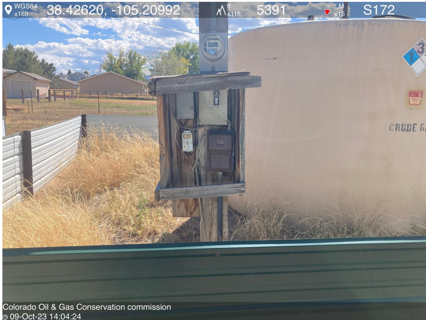
PHOTO 10: ELECTRIC PANEL IS APP. 3' FROM CRUDE OIL TANK BATTERY.
