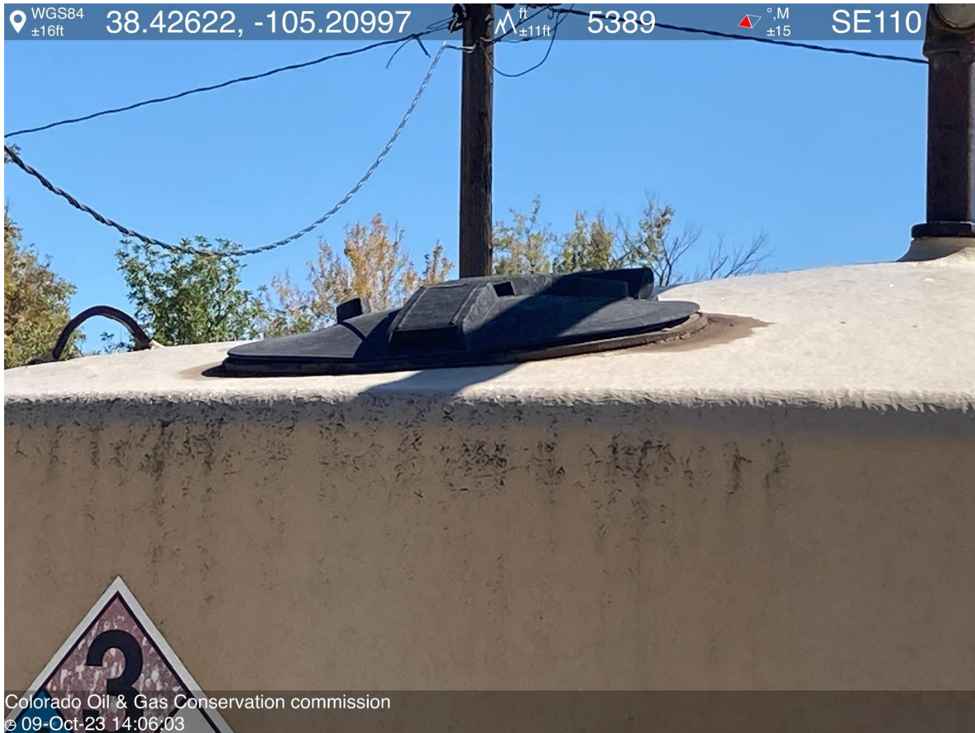
PHOTO 11: THERE APPEARS TO BE A RUBBER FLAP COVER ON TANK BATTERY WITH NO SAFETY VALVE INSTALLED ON TANK. Tanks will function as sealed and ventless with gas released only through a vapor control system or properly sized pressure relief valve. per Rule 608.a.(9). CA DATE 10-21-2023.
