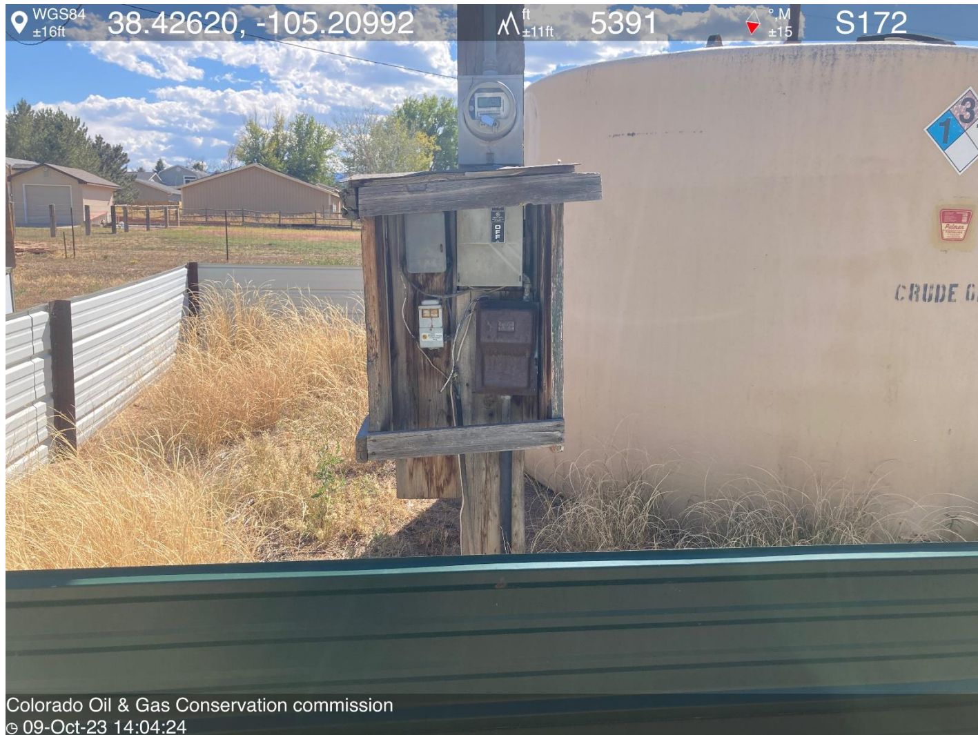
PHOTO 8: THERE ARE EXPOSED WIRE CONNECTIONS INSIDE WOOD ELECTRIC PANEL BOX. Securely fasten all valves, pipes, fittings, electric equipment and Production Facilities to ensure good mechanical condition, inspect at regular intervals and maintain in good mechanical condition per Rule 603.O(6) CA DATE 11-19-2023.
