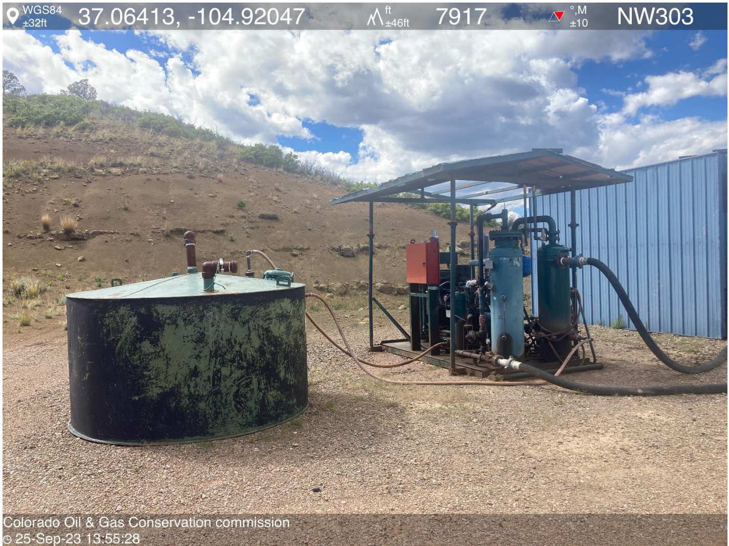
PHOTO 4: 30 BBLS PRODUCED WATER/USED OIL TANK.
