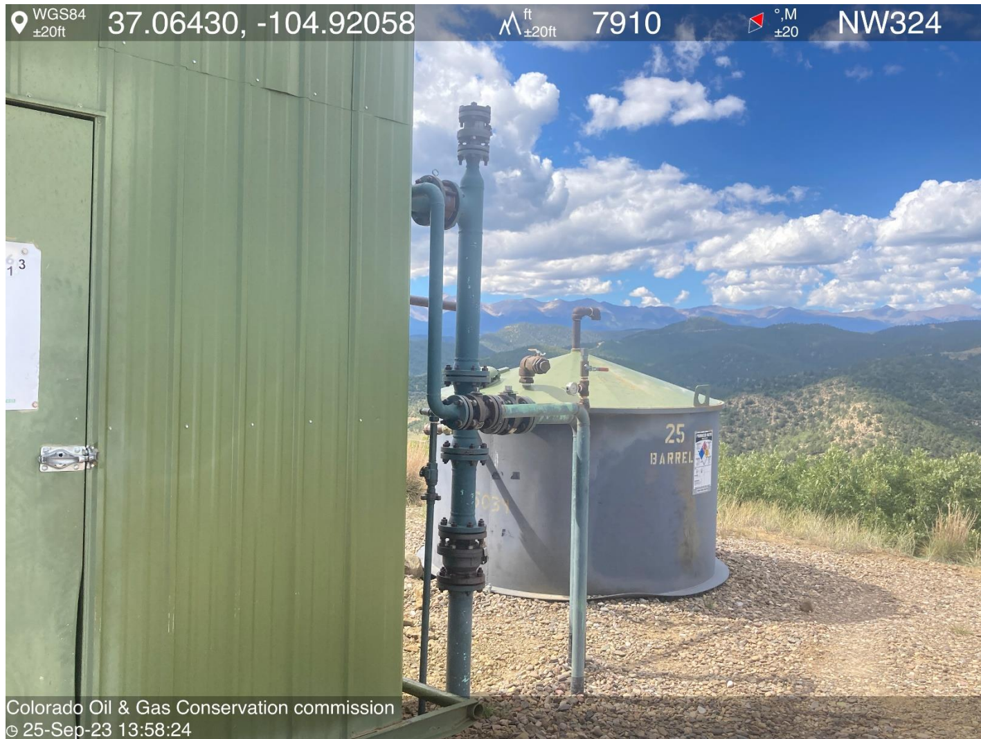
PHOTO 5: 25 BBLs PRODUCED WATER/USED OIL TANK.
