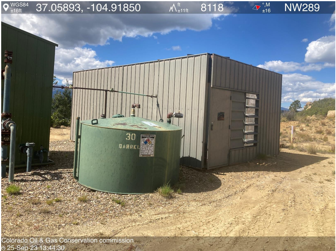
PHOTO 4: 30 BBLs PRODUCED WATER TANK & COMPRESSOR HOUSE.
