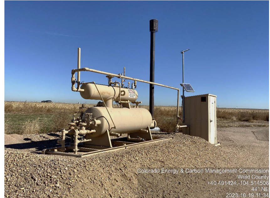
Photo #2 Holman 14-1 Battery site Inactive | Shut-down Separator(s)
