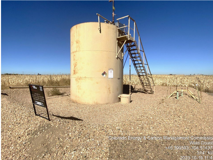
Photo #1 Holman 14-1 Battery site Inactive | Shut-down Tank(s): SE corner
