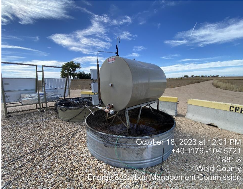
Missing sign/ Label contents and NFPA placard
