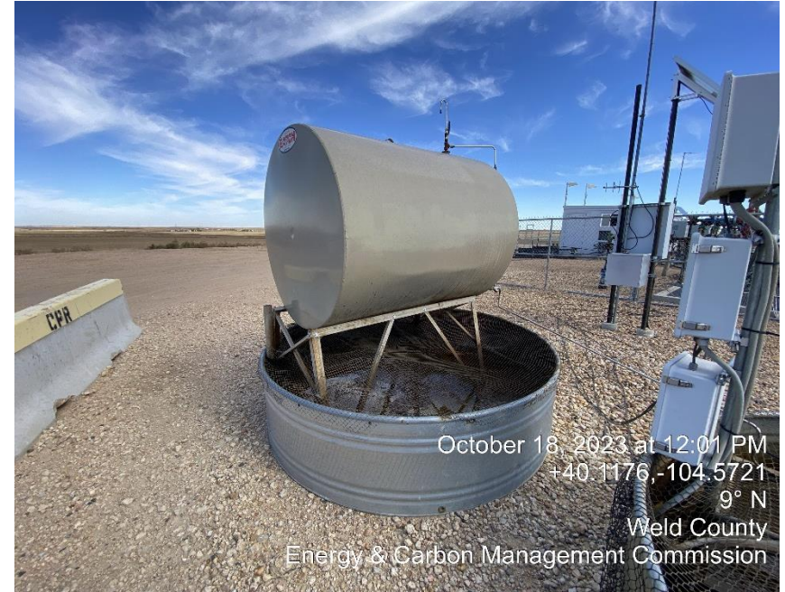
Missing sign/ Label contents and NFPA placard
