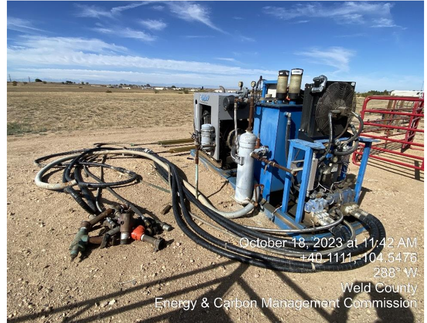
Prime Mover for Pumping unit
