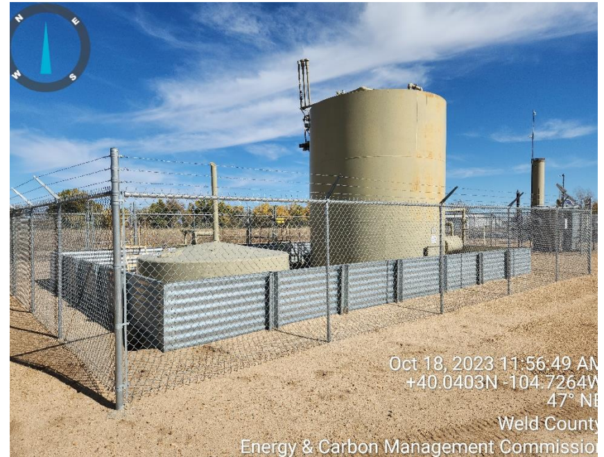
Photo 6 tank battery
