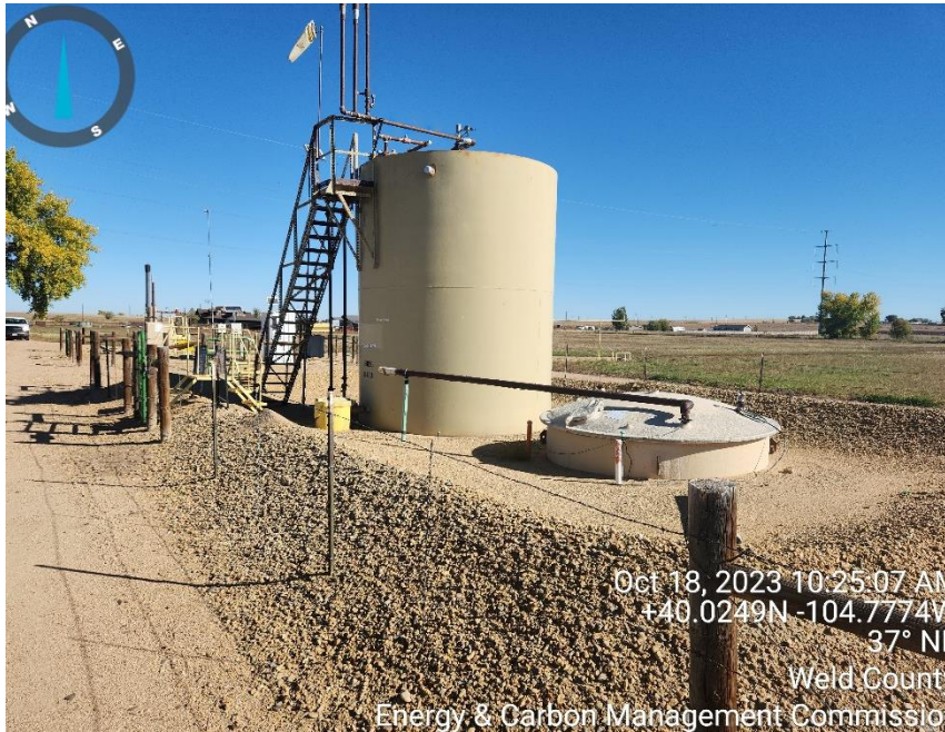
Photo 7 tank battery
