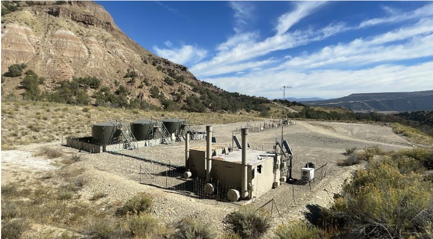
North West corner of location.
