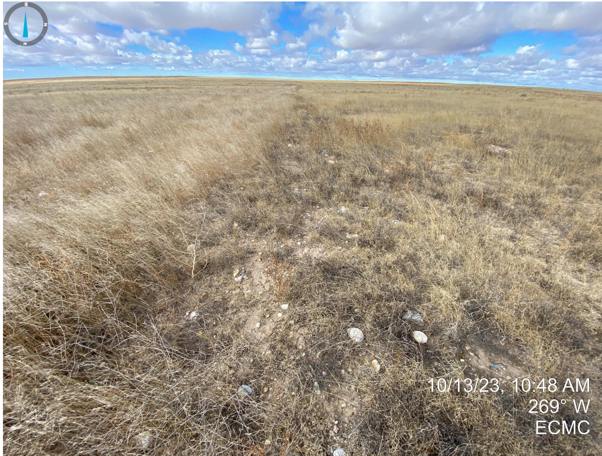
Photo 1. Taken from the access road. Road base material and cobble remain throughout the access road and requires removal. Photo is only an example as cobble and road base was observed throughout the entire access road.
