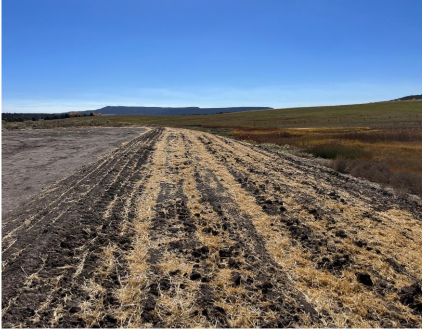
Photo #5 View of reseeded on west fill slopes.
