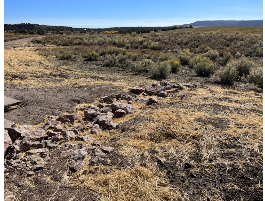
Photo #6 View of additional BMP installations.
