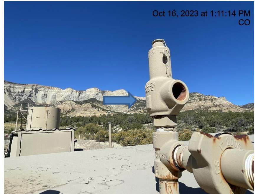
Photo # 2882 PRV lacks vent line
