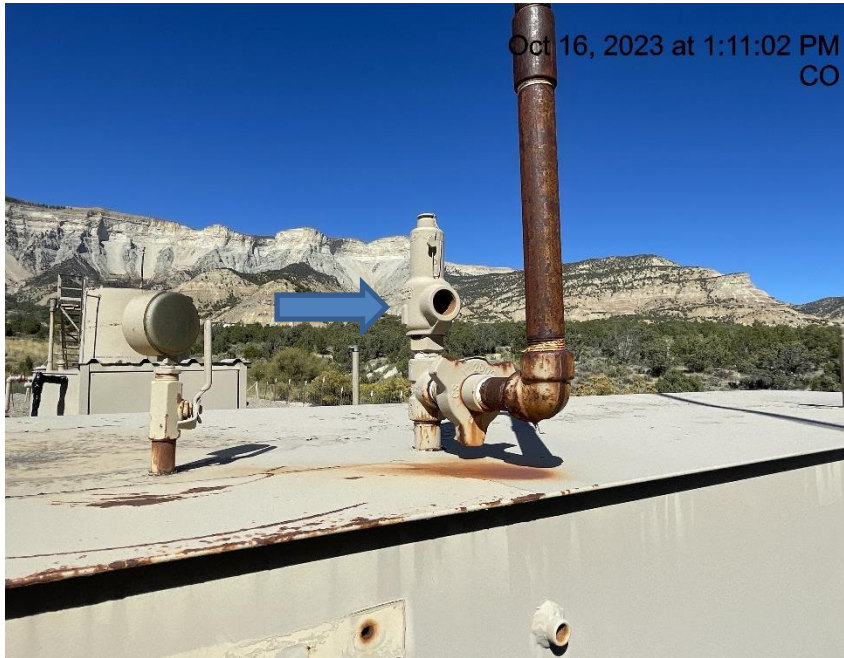
Photo # 2881 PRV lacks vent line
