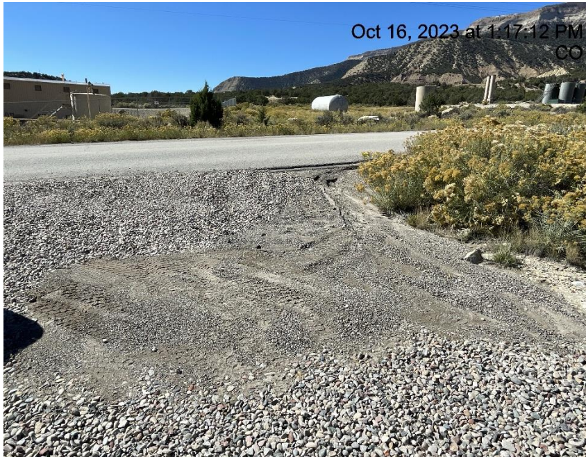
Photo # 2892 Sediment migrating onto gravel track pad/BMP needs maintenance
