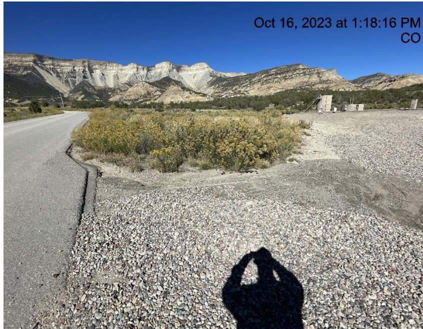
Photo # 2886 Sediment migrating onto gravel track pad/BMP needs maintenance
