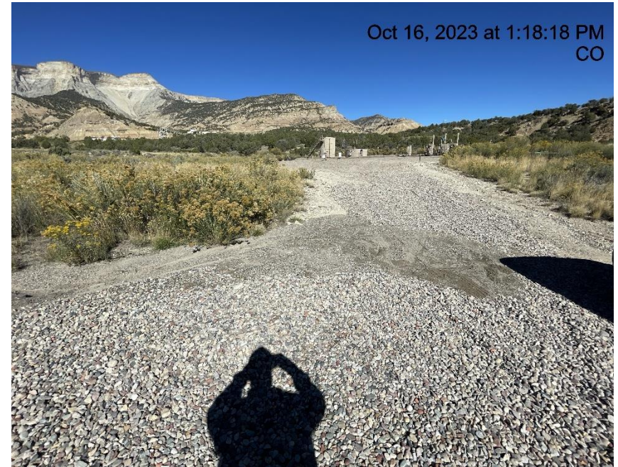
Photo # 2887 Sediment migrating onto gravel track pad/BMP needs maintenance
