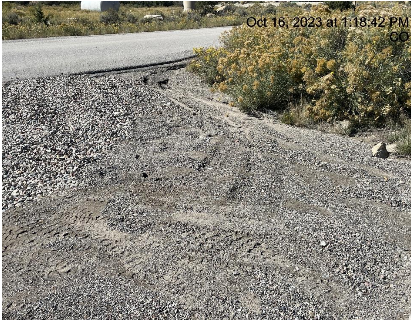
Photo # 2890 Sediment migrating onto gravel track pad/BMP needs maintenance
