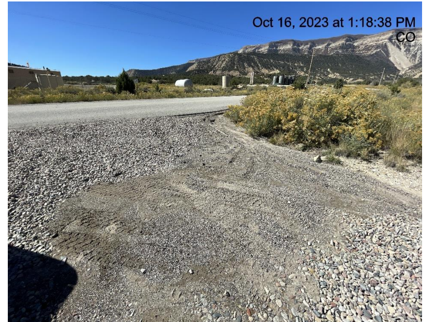
Photo # 2889 Sediment migrating onto gravel track pad/BMP needs maintenance
