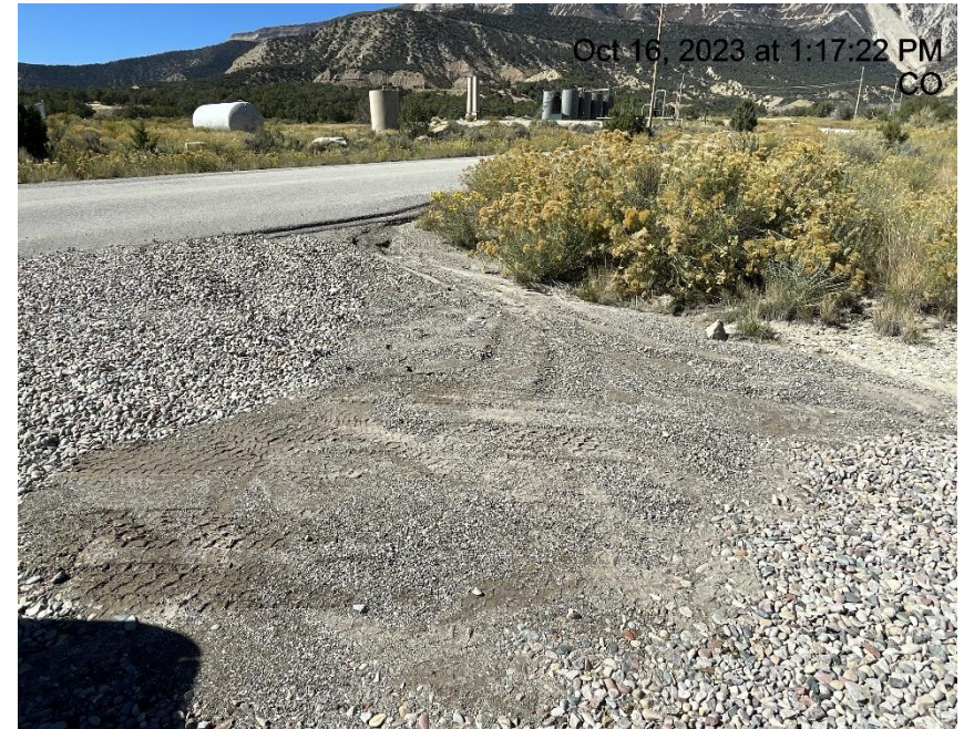
Photo # 2891 Sediment migrating onto gravel track pad/BMP needs maintenance
