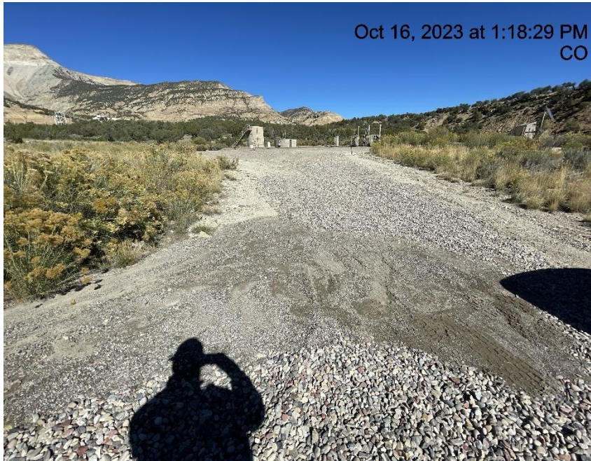
Photo # 2888 Sediment migrating onto gravel track pad/BMP needs maintenance
