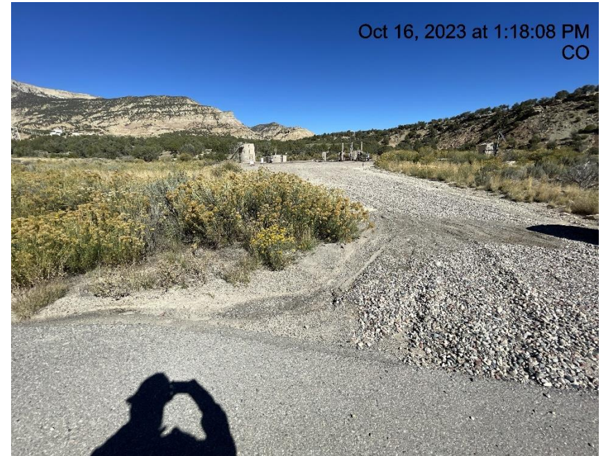
Photo # 2885 Sediment migrating onto gravel track pad/BMP needs maintenance
