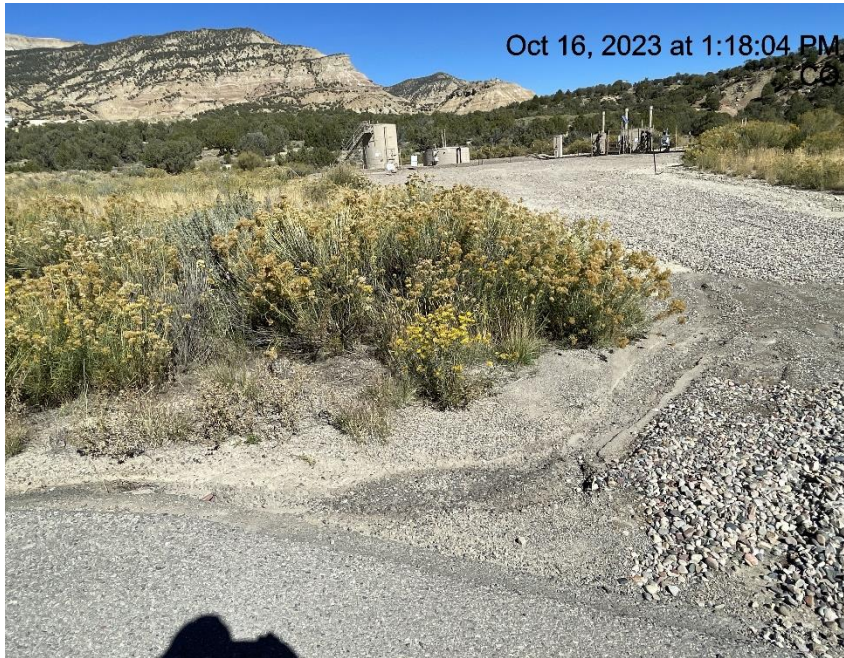
Photo # 2884 Sediment migrating onto gravel track pad/BMP needs maintenance
