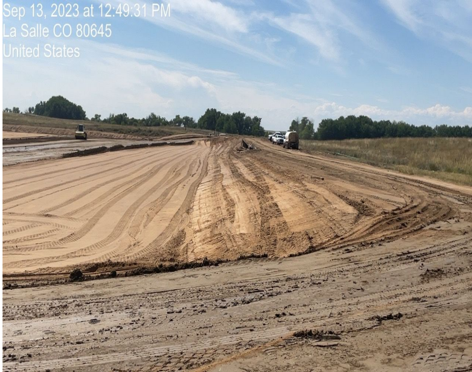
Photo 15. Photo taken of cut slope west side of pad and interior perimeter ditch. Photo taken facing south.
