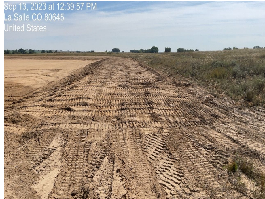
Photo 4. Photo taken of taken facing east of trackwalked topsoil stockpile on the south side of location.
