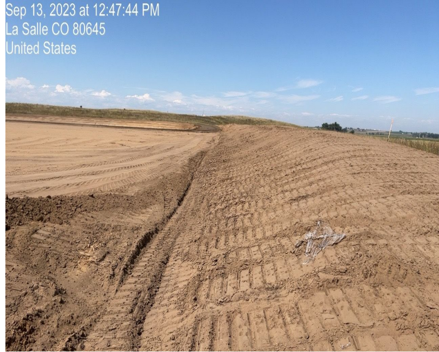
Photo 12. Photo taken of trackwalked topsoil stockpile and interior stormwater ditch on north side of location. Photo taken facing west.
