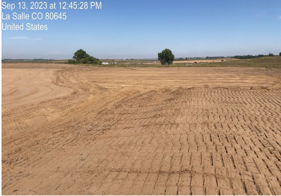
Photo 9. Photo taken of large sediment trap in northeast corner of pad. Photo taken facing north.
