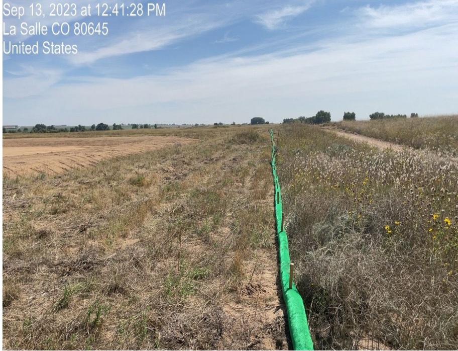
Photo 7. Photo taken of wattles at edge of disturbance on the south side of location. Photo taken facing east.
