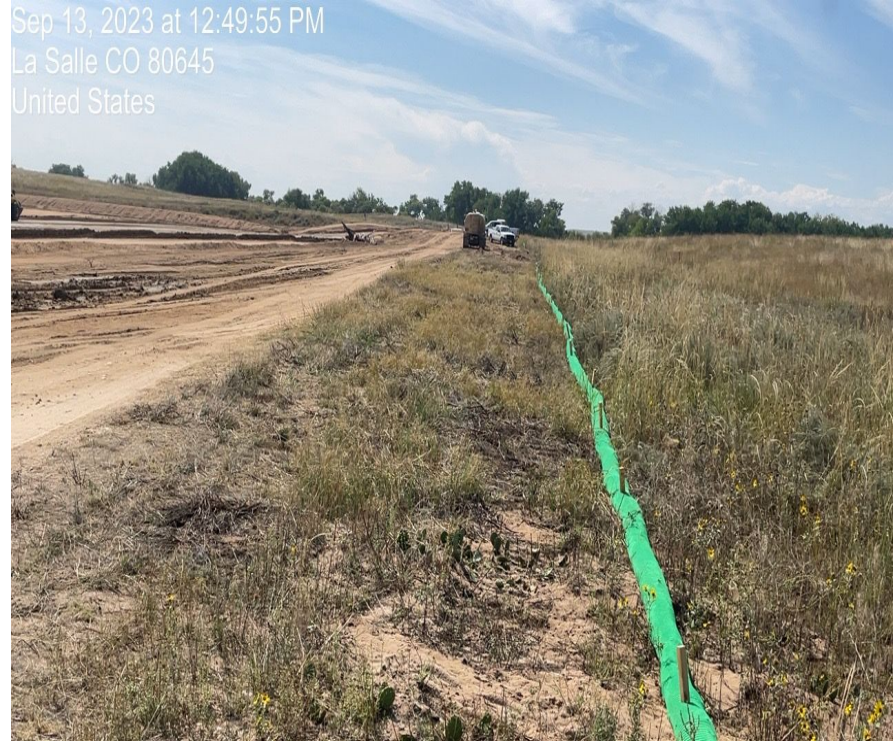
Photo 16. Photo taken photo taken of access road and wattles on west side of location. Photo taken facing south.
