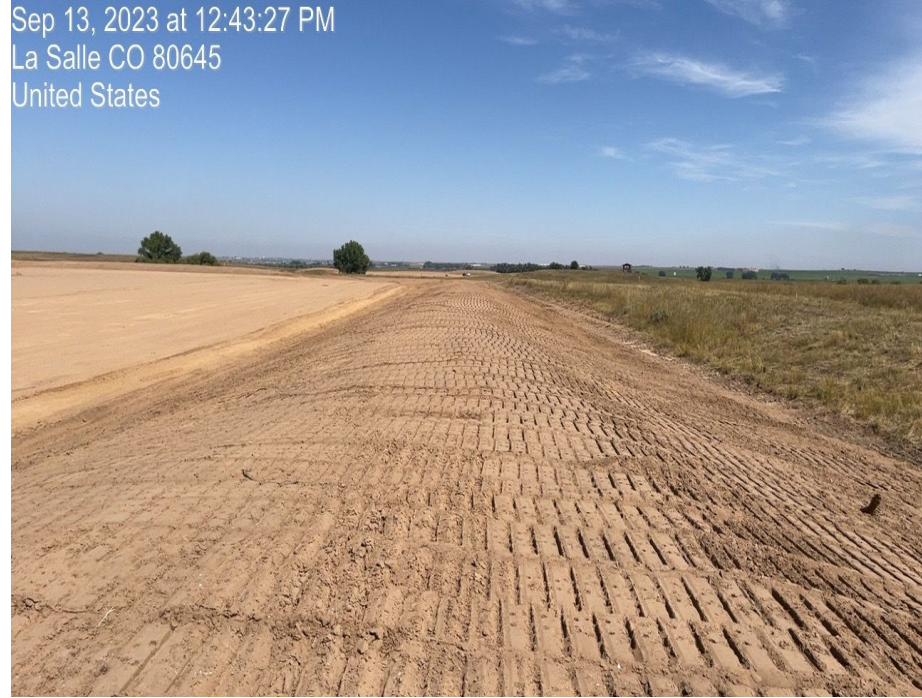
Photo 8. Photo taken of trackwalked topsoil stockpile on east side of pad. Photo taken facing North.
