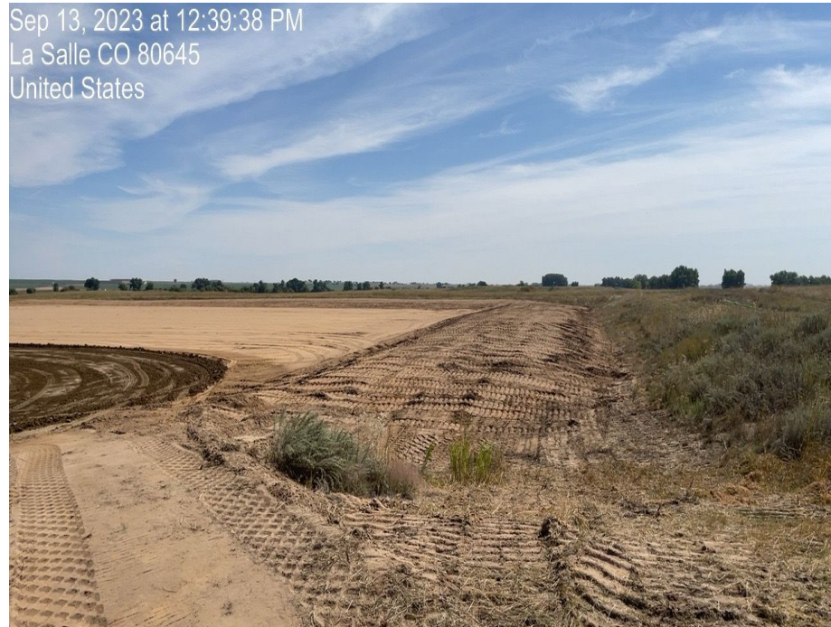
Photo 3. Photo taken of taken facing east of trackwalked topsoil stockpile on the south side of location.
