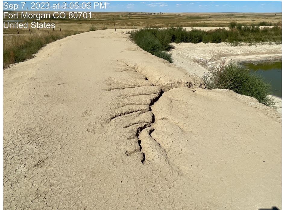
Photo 11. Photo taken facing northeast, of weeds (kochia) and stormwater caused erosion in un-stabilized pit berm leading into pit.
