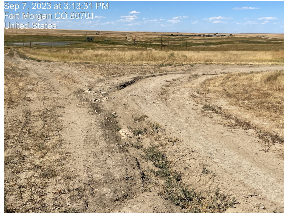
Photo 5. Photo taken facing north of access road to well head. Stormwater erosion caused gulying in the road way.
