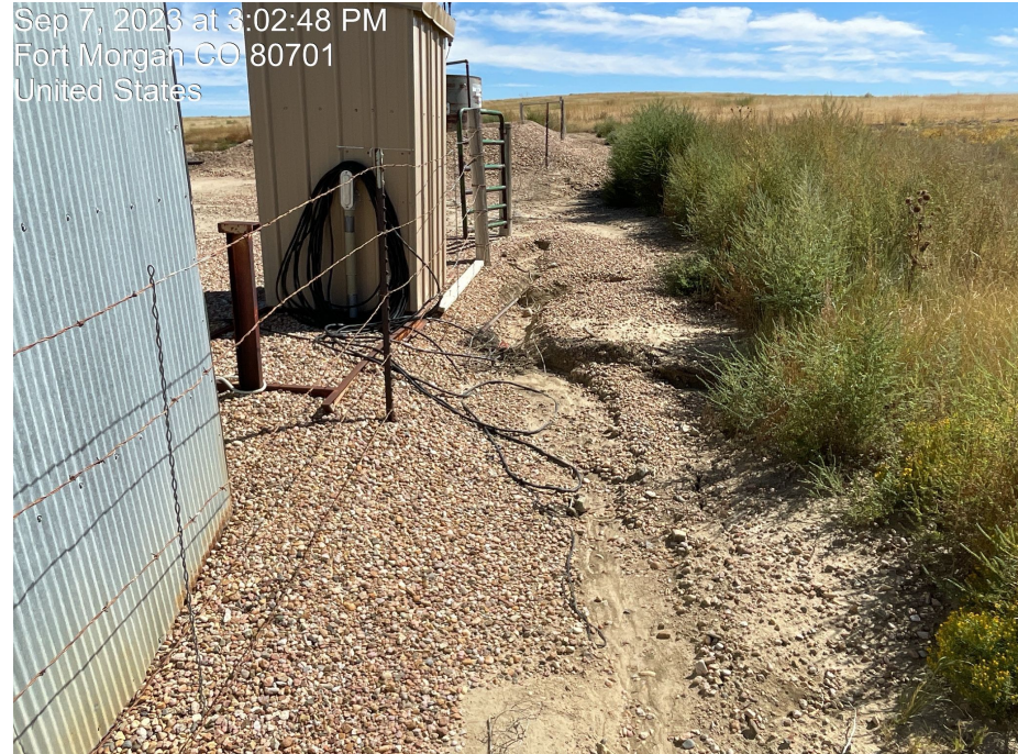
Photo 9. Photo taken facing south, of stormwater caused gully at gate to pit area.
