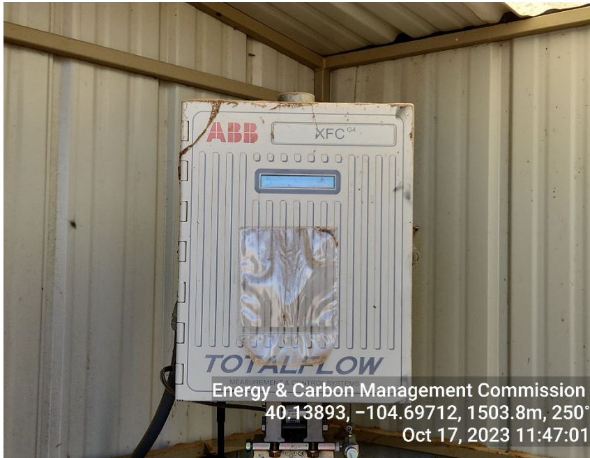
Photo 17: Gas meter disconnected
