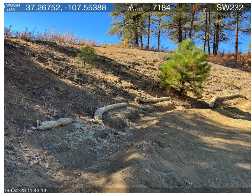
Photo #2. Corrective action completed. BMPs installed. BMPs not effective.
