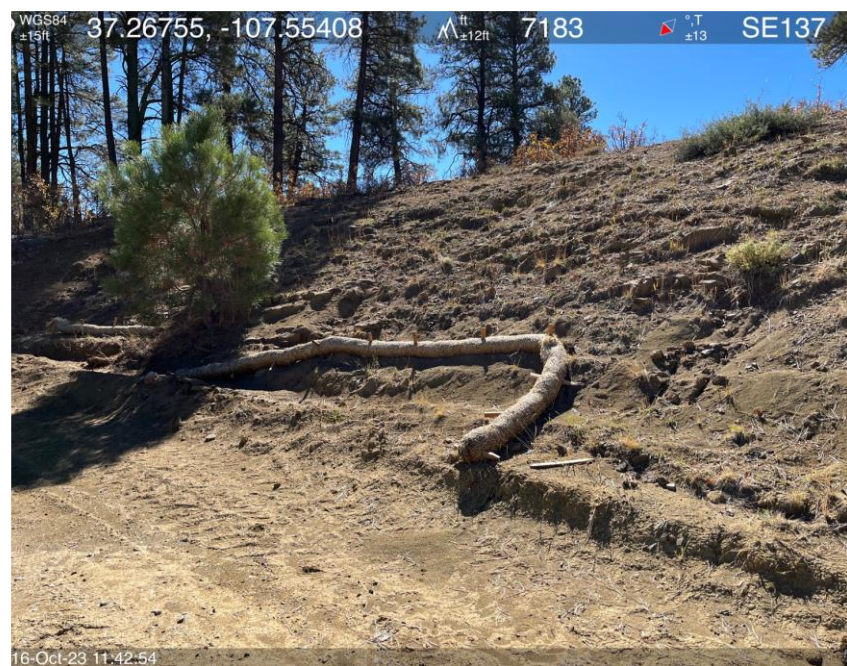
Photo #4. BMPs installed, not effective.
