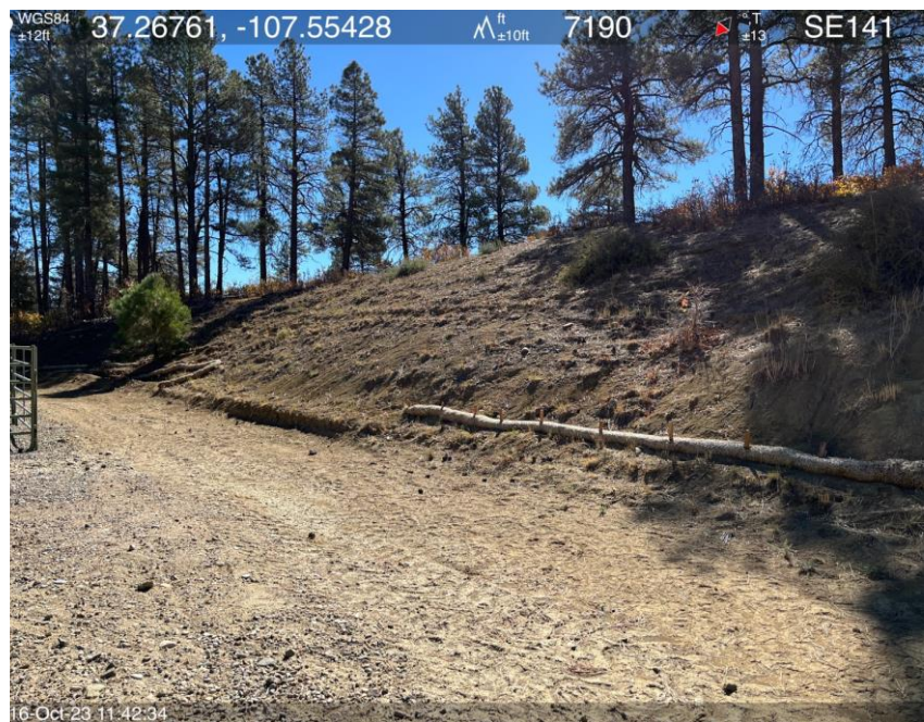
Photo #3. BMPs installed, not completed.
