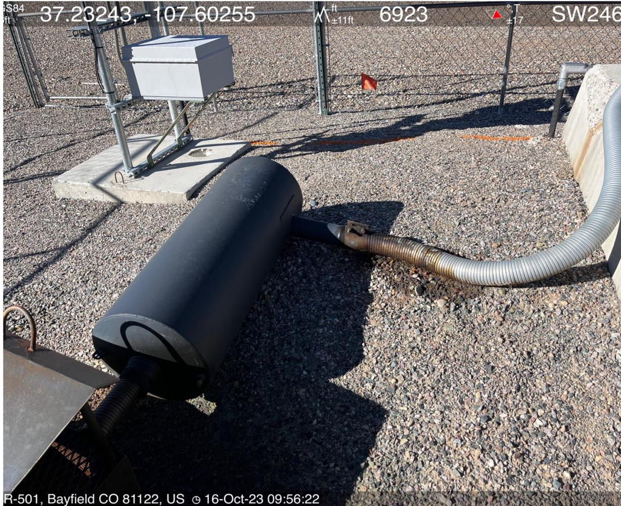
Photo #7 View of impacted material at muffler.
