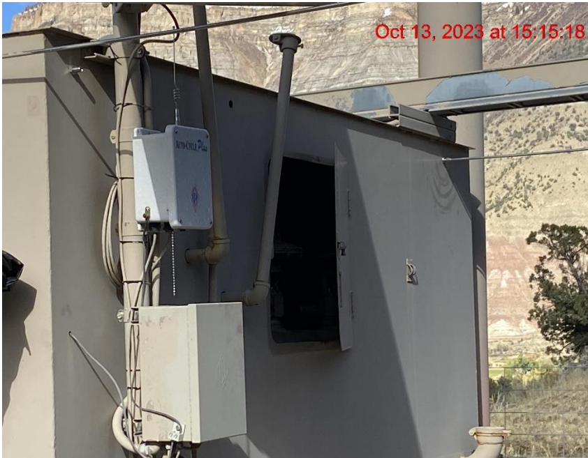
Unsecured Hatch on Separator– Photo #06931
