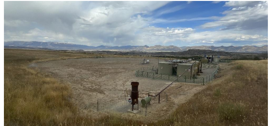
South East corner of location.
