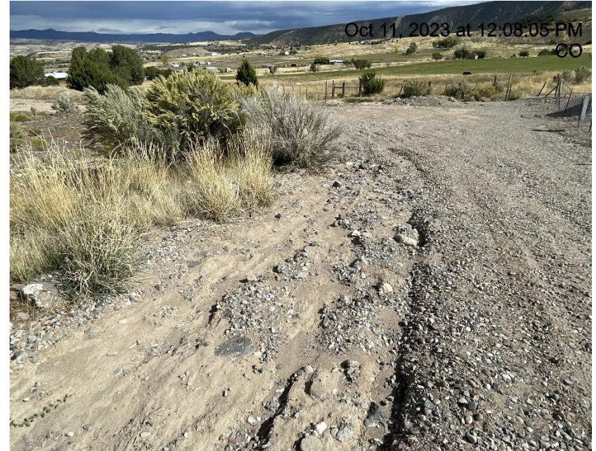
Photo # 2428 Erosion & transport of sediment on lease road near entrance to location
