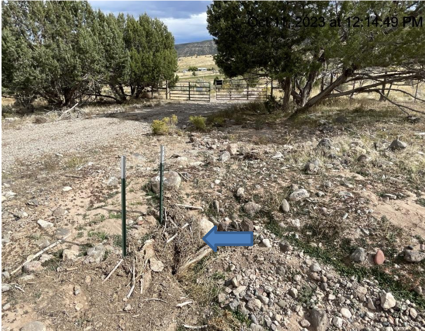
Photo # 2429 Culvert on lease road needs maintenance
