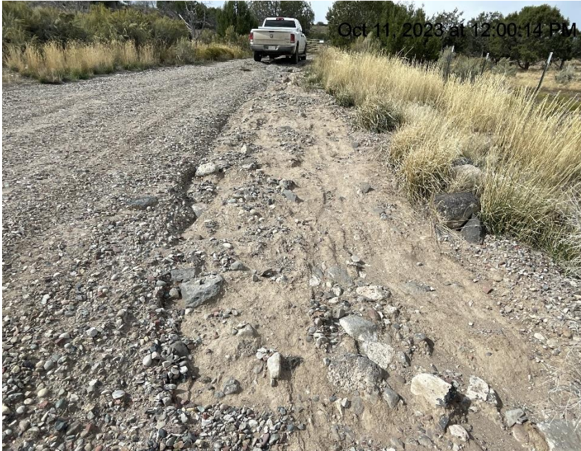
Photo # 2427 Erosion & transport of sediment on lease road near entrance to location
