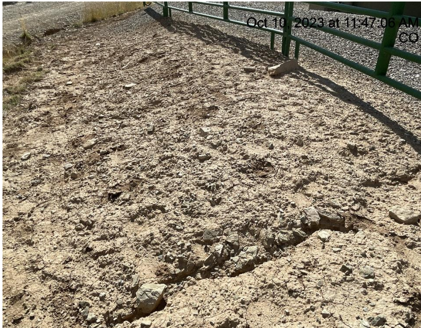
Photo # 2224 Erosion & transport of sediment on slope (SE side of location behind tank battery containment)
