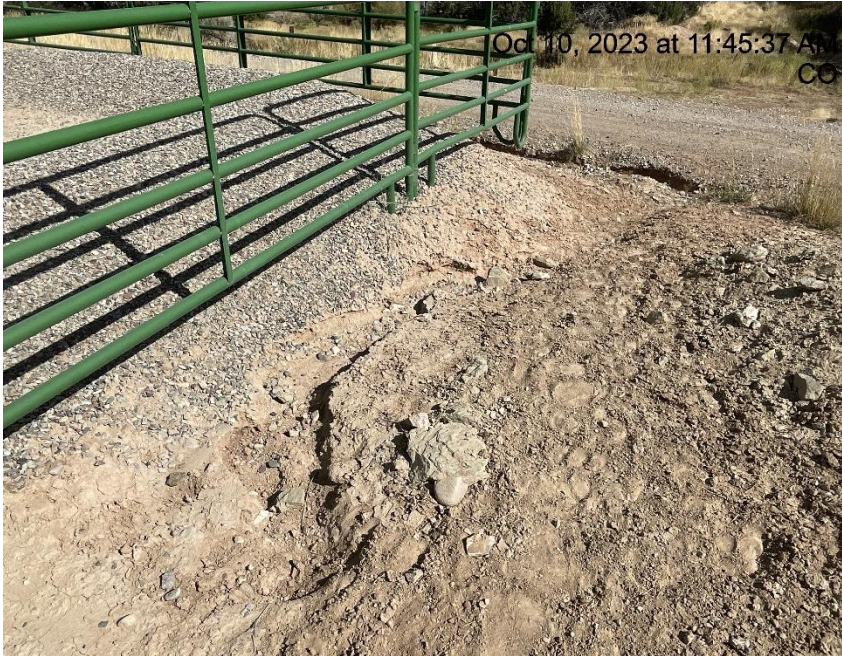
Photo # 2220 Erosion & transport of sediment off location/insufficient BMP's (SE corner of location near tank battery containment)
