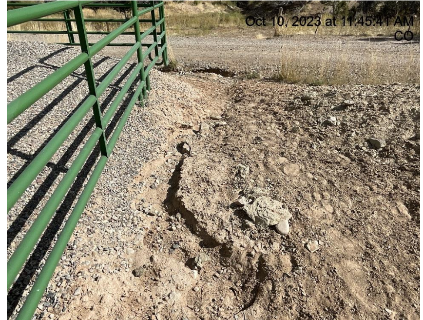
Photo # 2221 Erosion & transport of sediment off location/insufficient BMP's (SE corner of location near tank battery containment)
