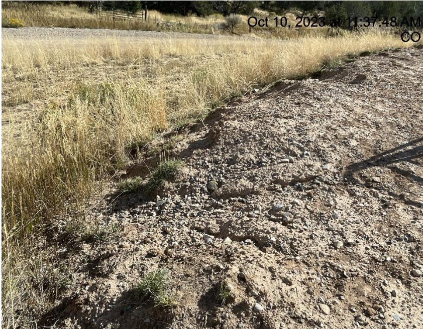
Photo # 2228 Erosion & transport of sediment off location (N/NE side of location in multiple areas)
