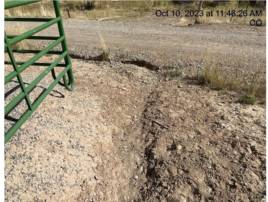
Photo # 2223 Erosion & transport of sediment off location/insufficient BMP's (SE corner of location near tank battery containment)
