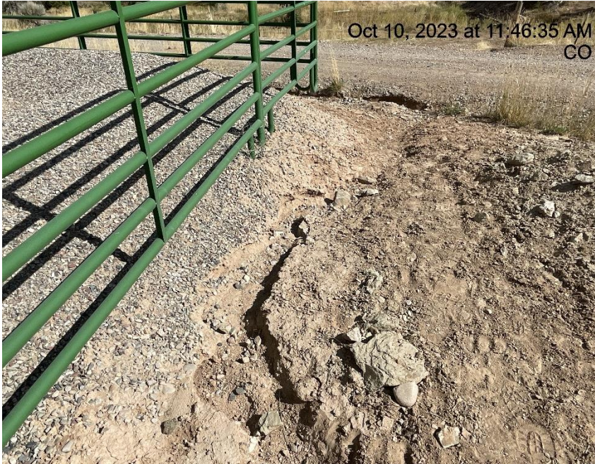
Photo # 2222 Erosion & transport of sediment off location/insufficient BMP's (SE corner of location near tank battery containment)
