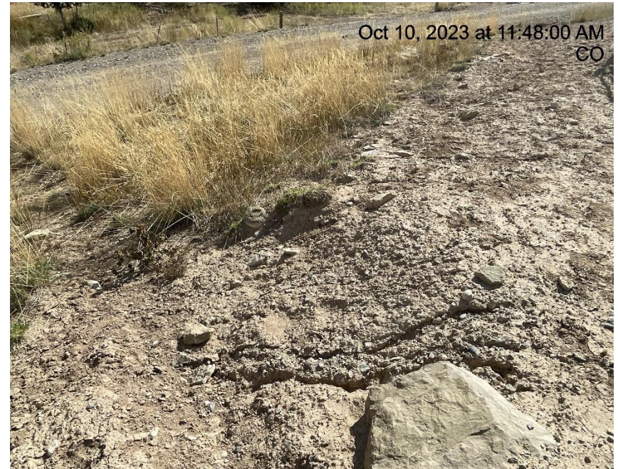
Photo # 2227 Erosion & transport of sediment off location/insufficient BMP's (SE side of location behind tank battery containment)
