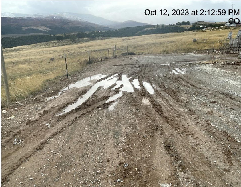
Photo # 2740 Lack of stabilization/compaction
