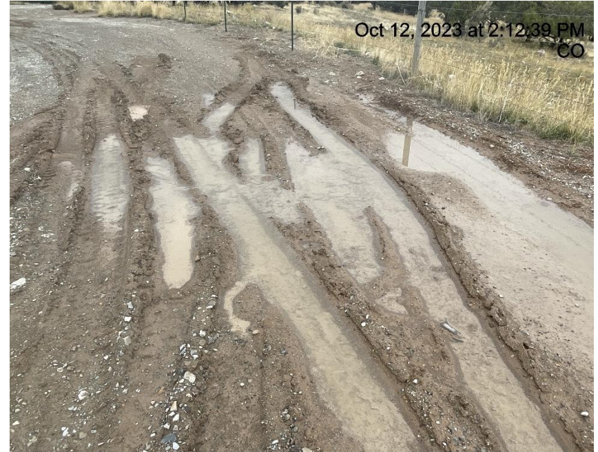
Photo # 2741 Lack of stabilization/compaction
