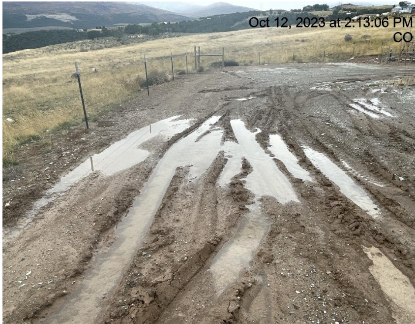
Photo # 2742 Lack of stabilization/compaction
