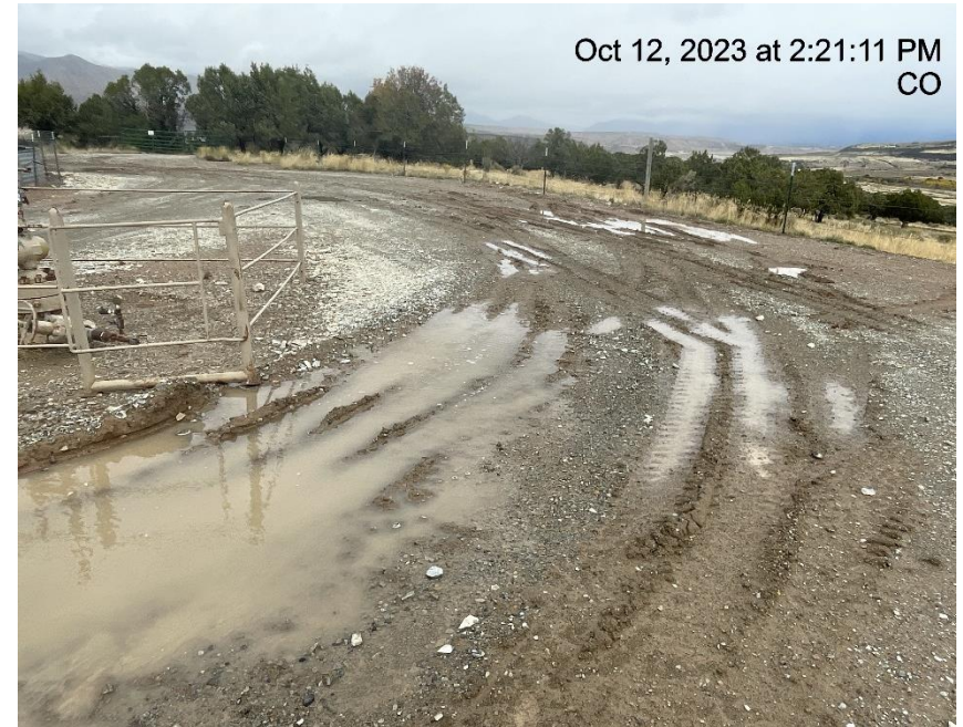
Photo # 2745 Lack of stabilization/compaction
