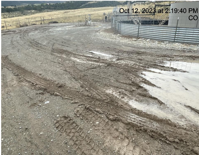
Photo # 2746 Lack of stabilization/compaction
