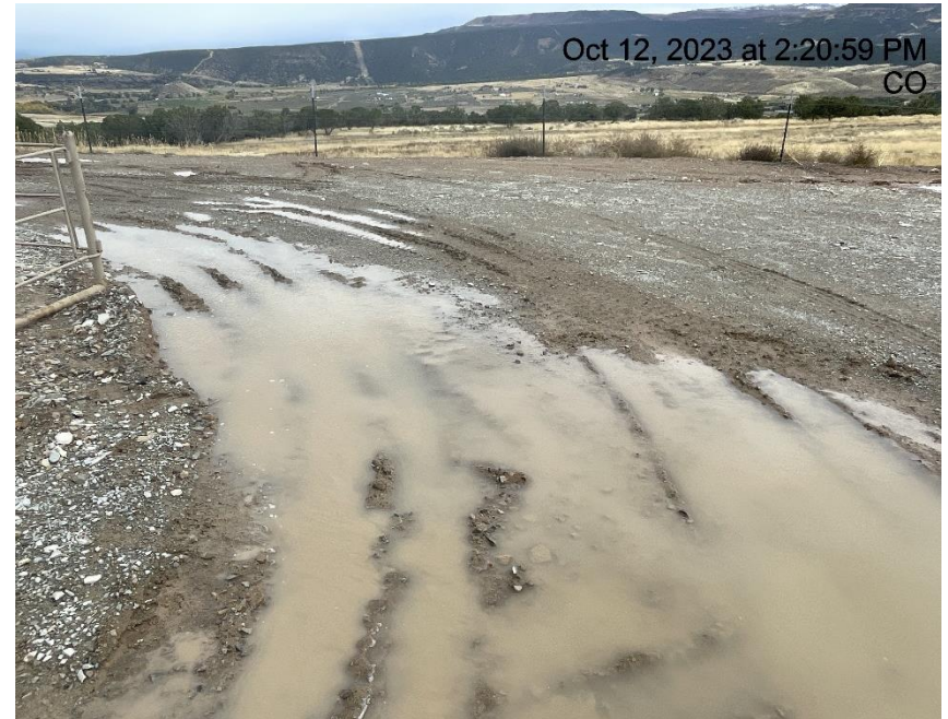
Photo # 2743 Lack of stabilization/compaction
