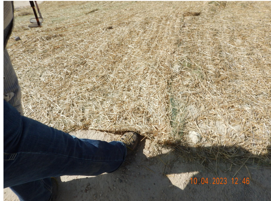
Photo 10. Photo of erosion control blanket that has not been properly trenched.
