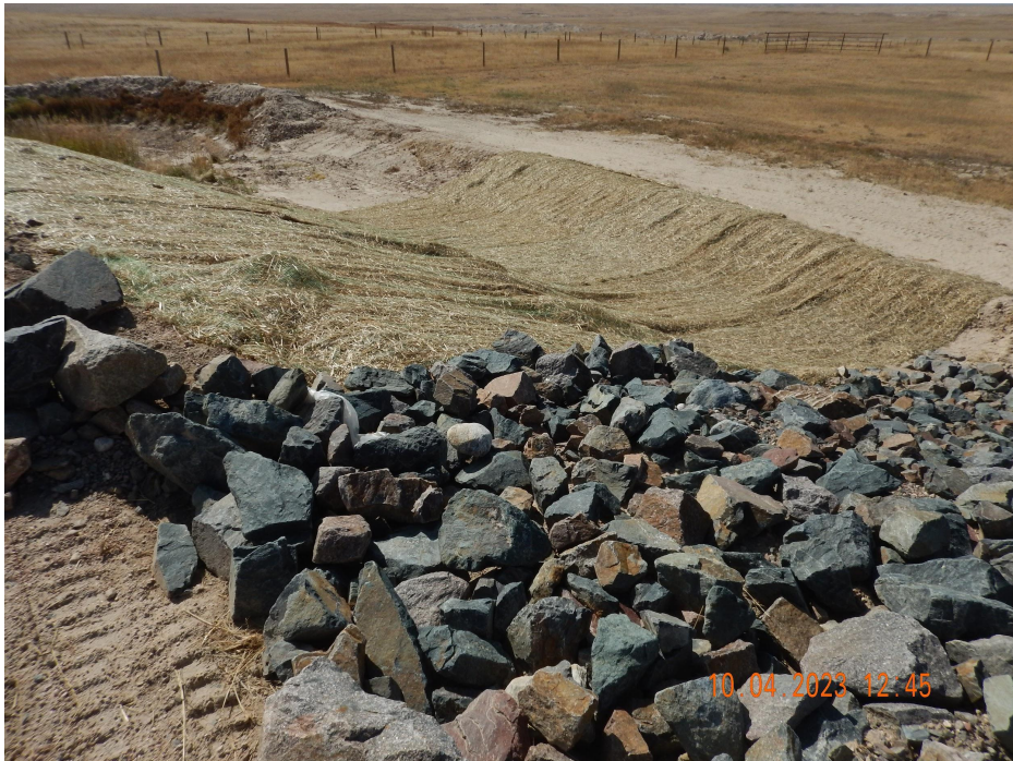
Photo 9. Photo taken from the southwestern well pad, facing Southwest. Photo illustrates erosion control blankets have been installed but were not properly trenched- see Photo 10.
