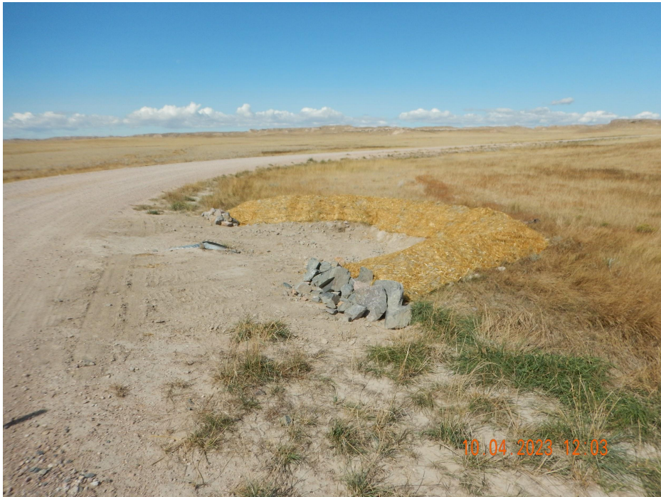
Photo 3. Photo taken from a portion of the access road, facing Northwest. Photo illustrates stormwater BMP repairs along the inlet area of a culvert crossing. The BMP is an improvement from the previous condition but there are additional engineering practices that shall be implemented- see Photo 4.
