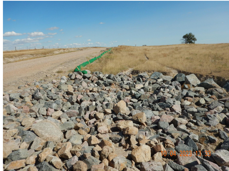
Photo 12. Photo taken from Geary Creek, facing East. Photo illustrates the Operator has installed riprap into the eastern channel and added filtrex wattles.
