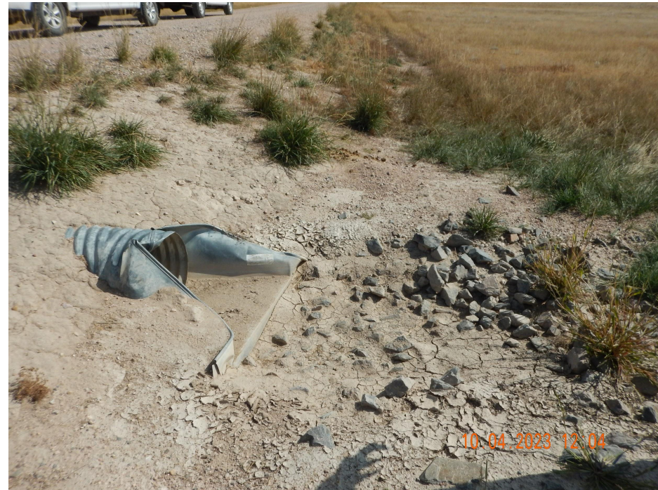
Photo 4. Photo taken from the outlet of the culvert, facing South. The outlet area of the culvert lacks sufficient stabilization. Sediment discharge was observed out into the adjacent areas beyond the outlet area.
