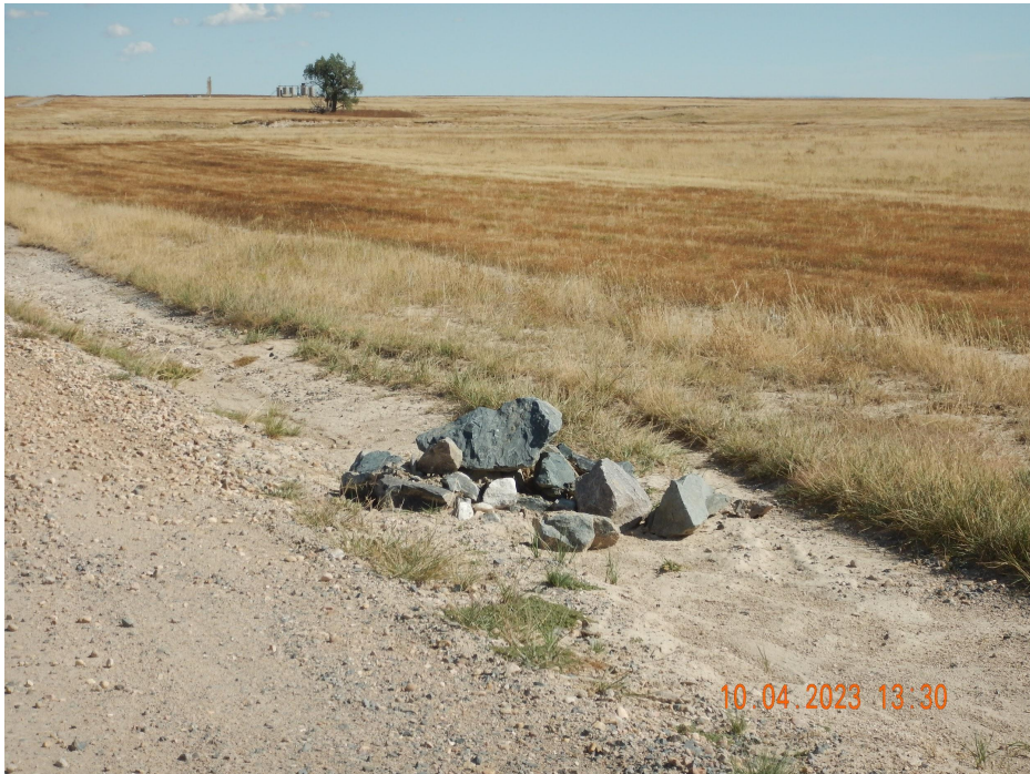
Photo 1. Photo taken from a portion of the access road, facing East. Photo illustrates a check dam BMP that has not been installed per good engineering practices. It appears rocks were dumped in the ditch without being properly keyed in, which means the crest and weir are not to specifications. Also, there does not appear to be any geotextile under the check dam.
