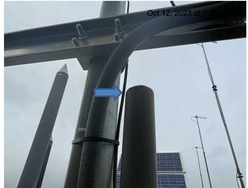
Photo # 2702 SR 411-9 rupture disk vent line lacks cap
