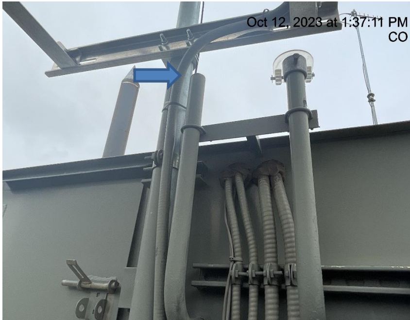
Photo # 2701 SR 411-9 rupture disk vent line lacks cap
