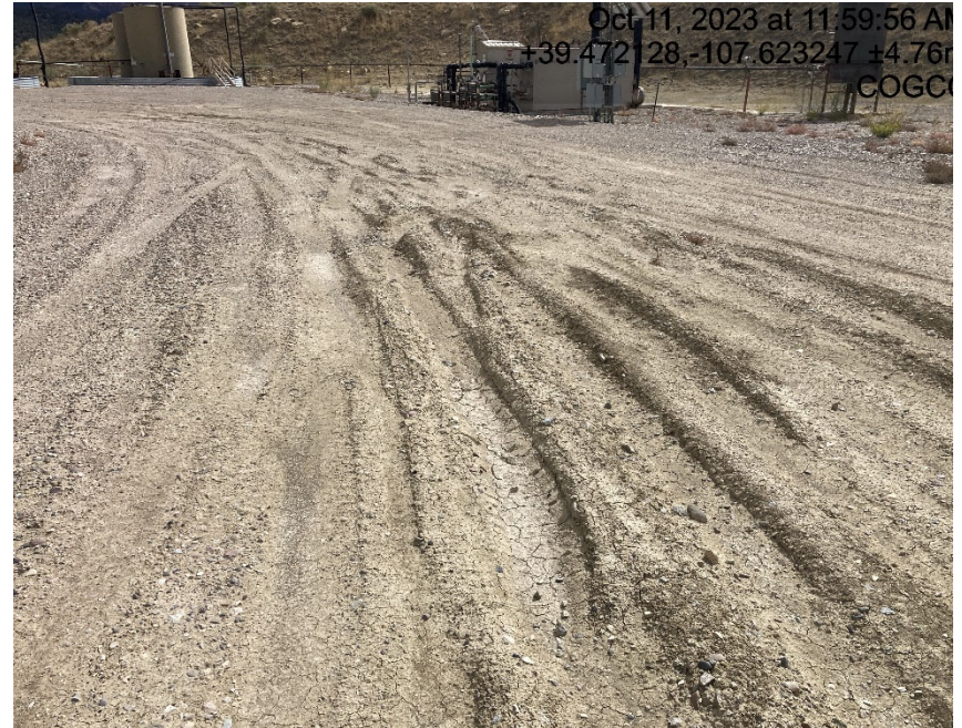
Lack of stabilization/compaction
