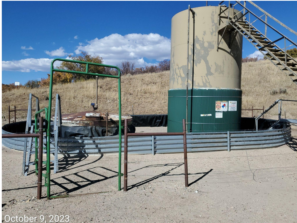
Photo 8: Tank battery facility, north end of the Location. Tank battery signage not posted pursuant to Rule 605.e
