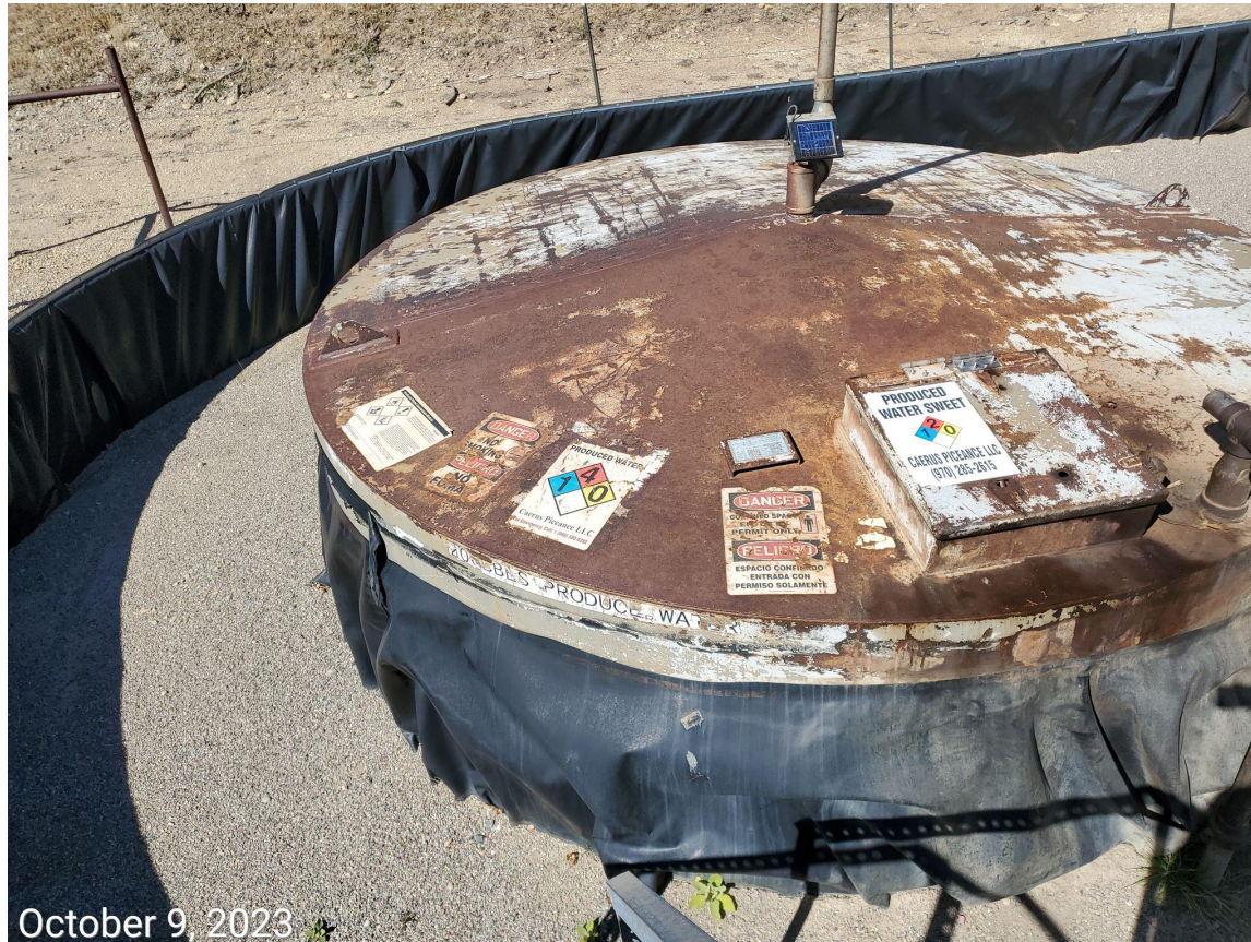
Photo 9: Photo taken from the tank battery facility. Capacity labeling on tank no longer legible.
