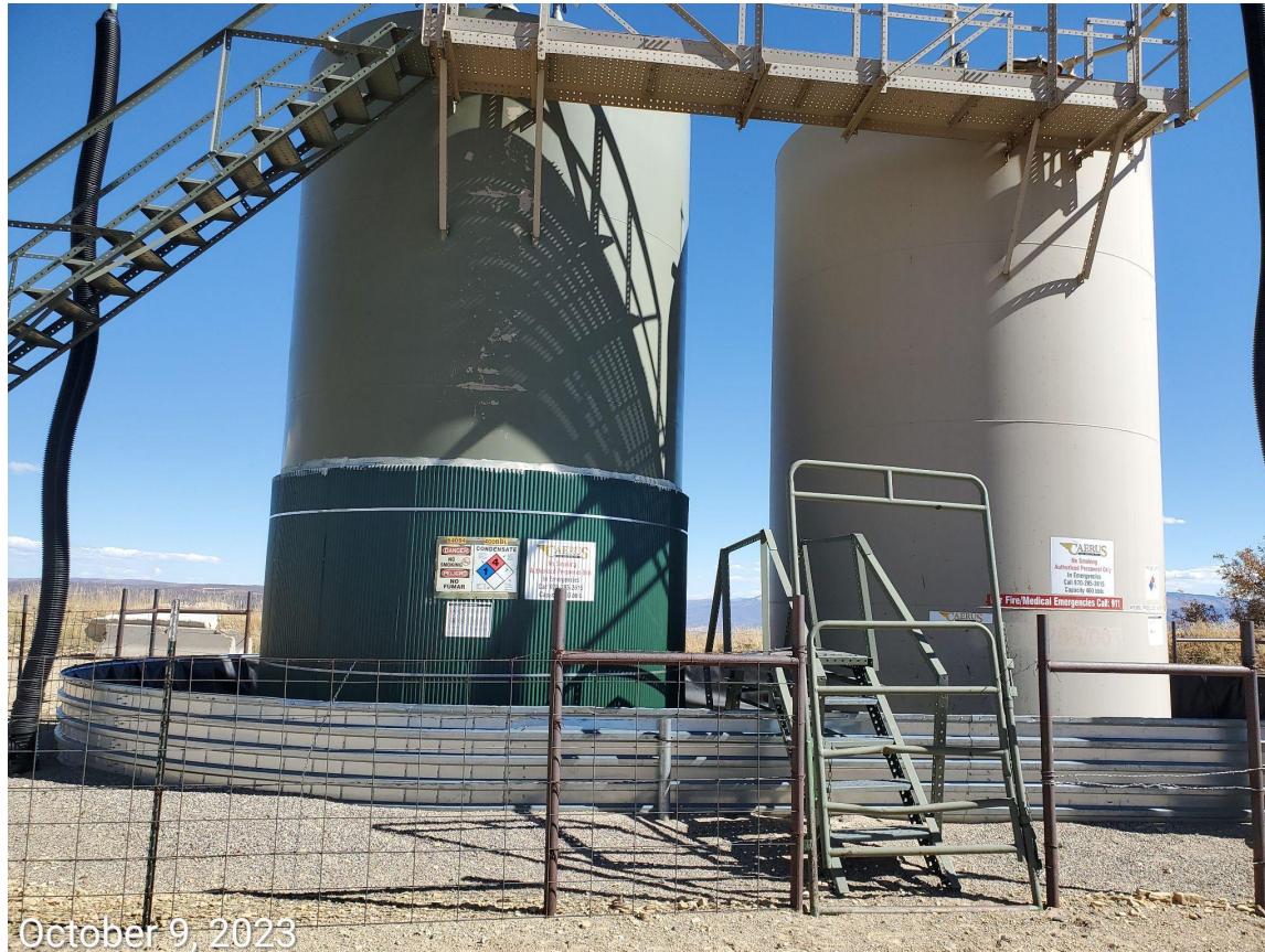
Photo 6: Tank battery facility, south end of the Location. Tank battery signage not posted pursuant to Rule 605.e
