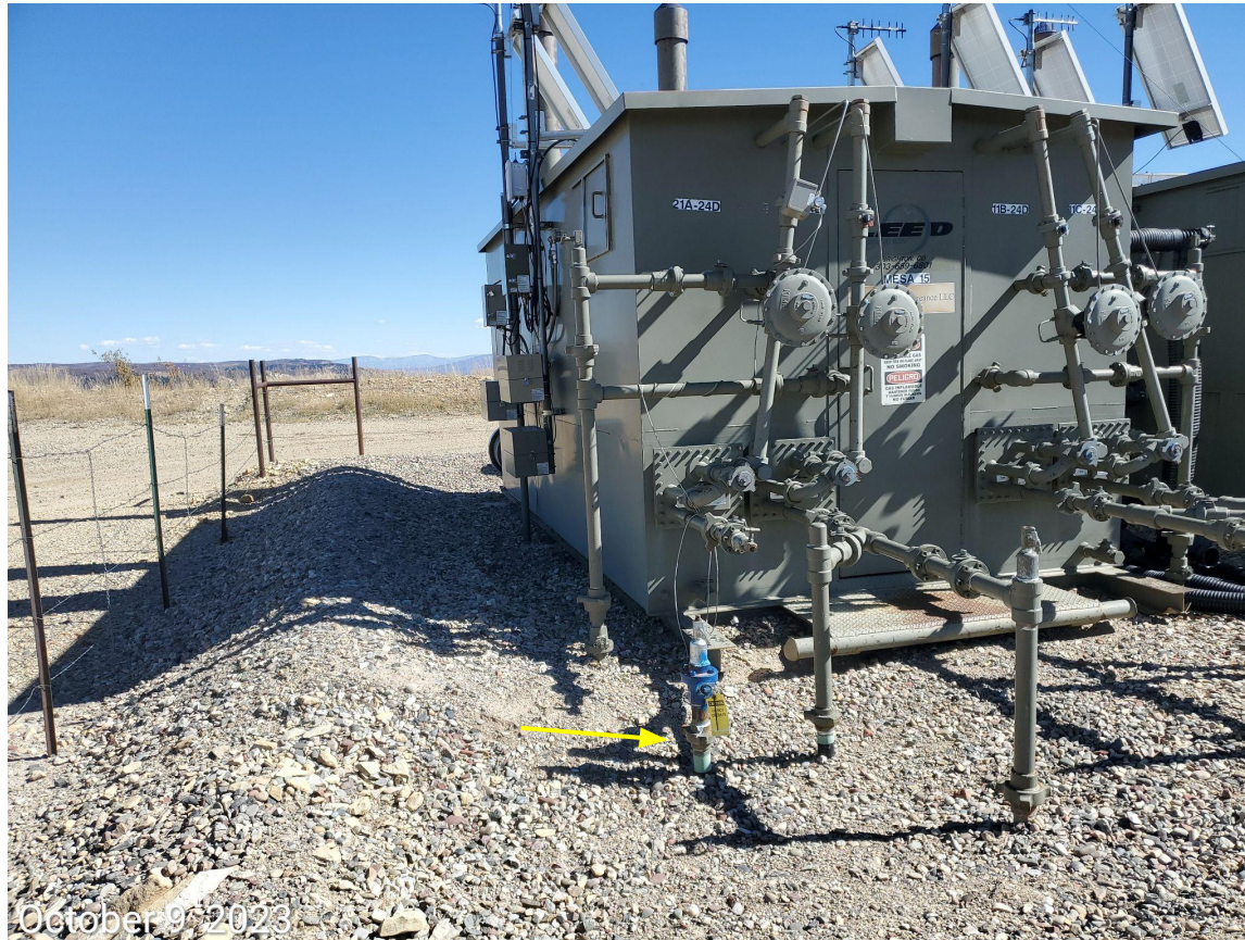
Photo 5: Photo taken from the separator equipment, facing east. Photo shows flowline riser associated with the abandoned 21A-24D well remaining on the Location.
