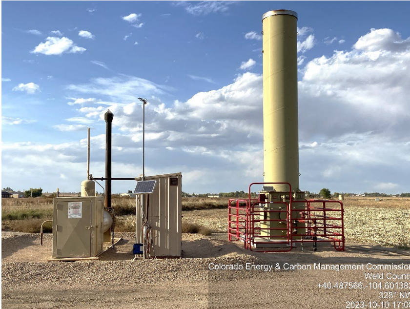
Photo #3 Heldt 12-18 Battery site Active Separator(s), ECD(s)
