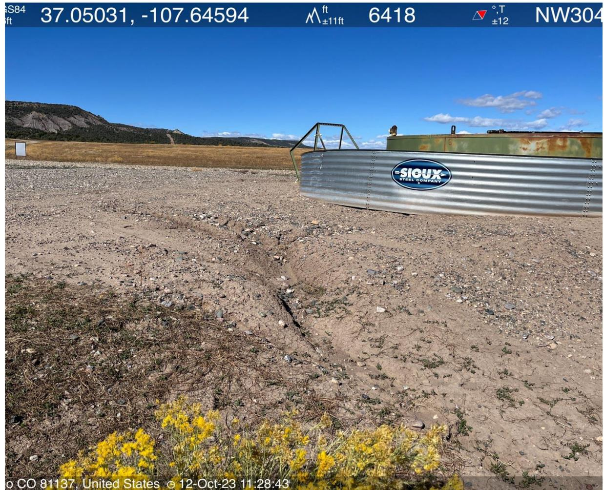
Photo #5 View of erosion and sediment migration.
