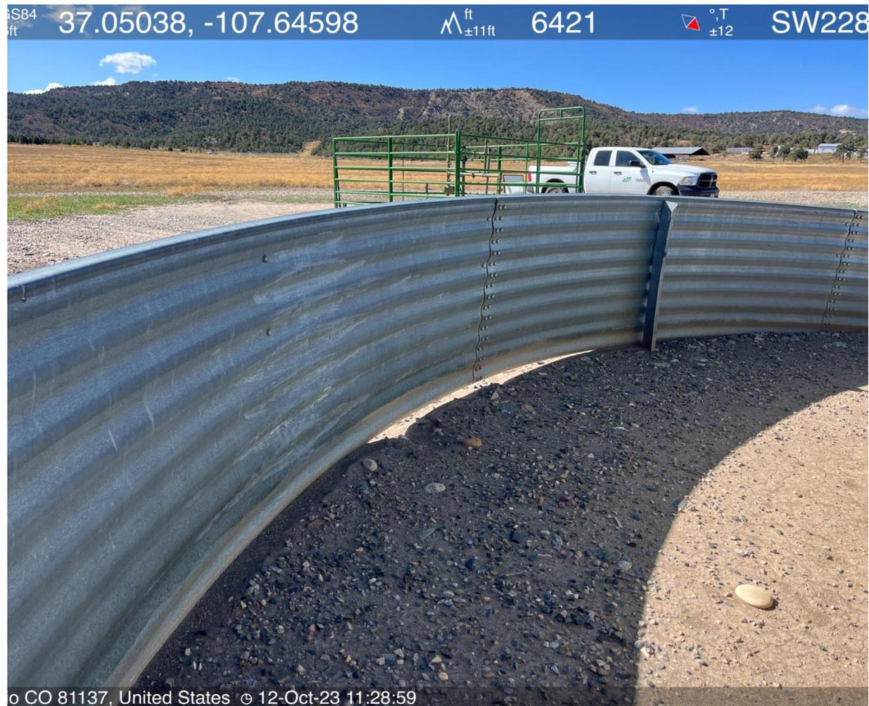
Photo #6 View of non-impervious tank containment.
