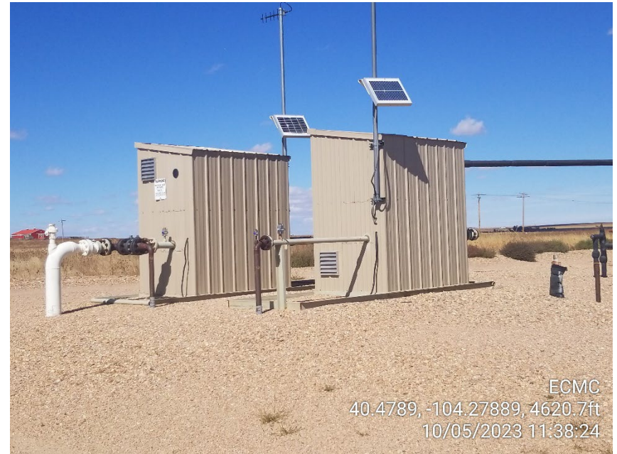
Photo 6 – Gas Meter Houses
