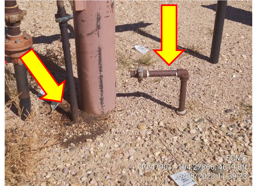
Photo 10 – Stained Soil and Unmarked Riser
