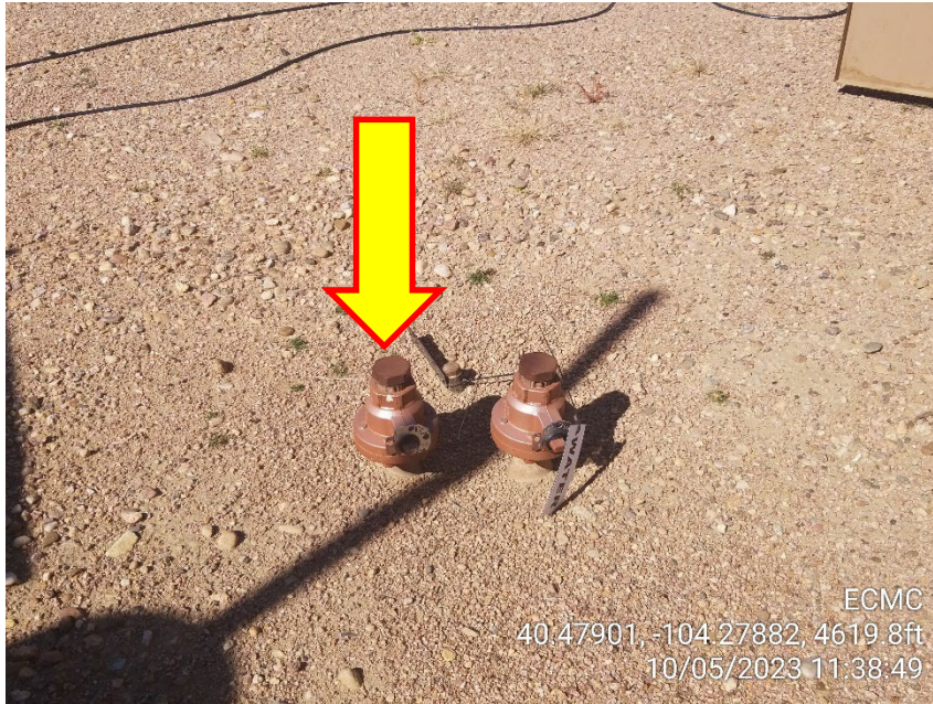
Photo 7 – Unmarked Riser at Separators
