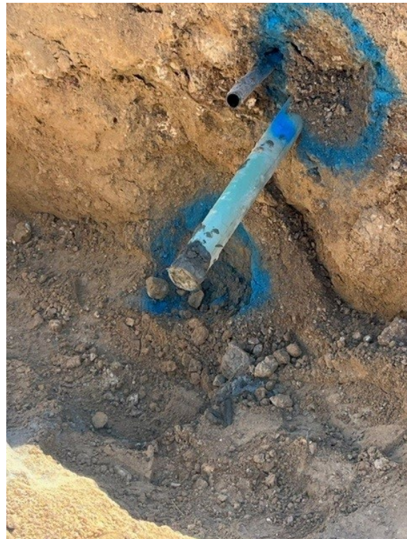
Riser cut, line packed W cement, Facing South
