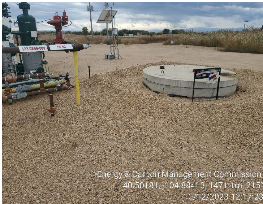
60 bbls concrete compressor vault berm
