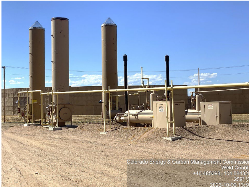
Photo #3 Foos A18-23 Battery site Inactive / Shut-down Separator(s), ECD(s)
