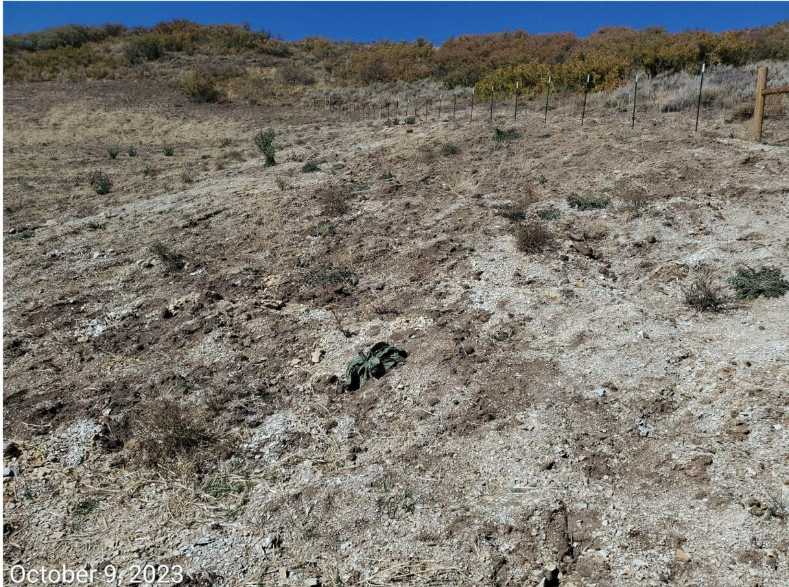
**Photo 5:** Photo taken from the northwest end of the Location, facing west. Photo example showing areas where mulch had not been uniformly applied and/or anchored; mulch on Location has been blown onto the soil surface, and was not observed to be anchored mechanically (such as crimping or a tackifier).
