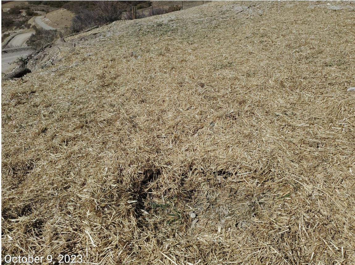
**Photo 14:** Photos example showing downslope areas where mulch has either been applied too thickly, or is accumulating due to lack of anchoring in conjunction with wind/water/gravity. Mulch was ~6 inches thick in such areas.
