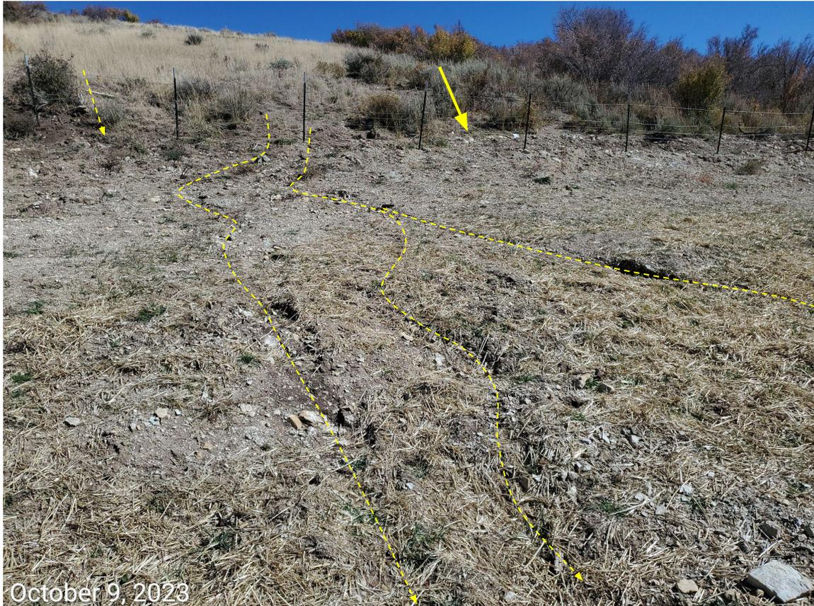
**Photo 9:** Photo example showing erosion degradation is becoming apparent. Perimeter control measures to manage runoff have not been implemented. Yellow arrows represent flow direction; lines outline erosion.
