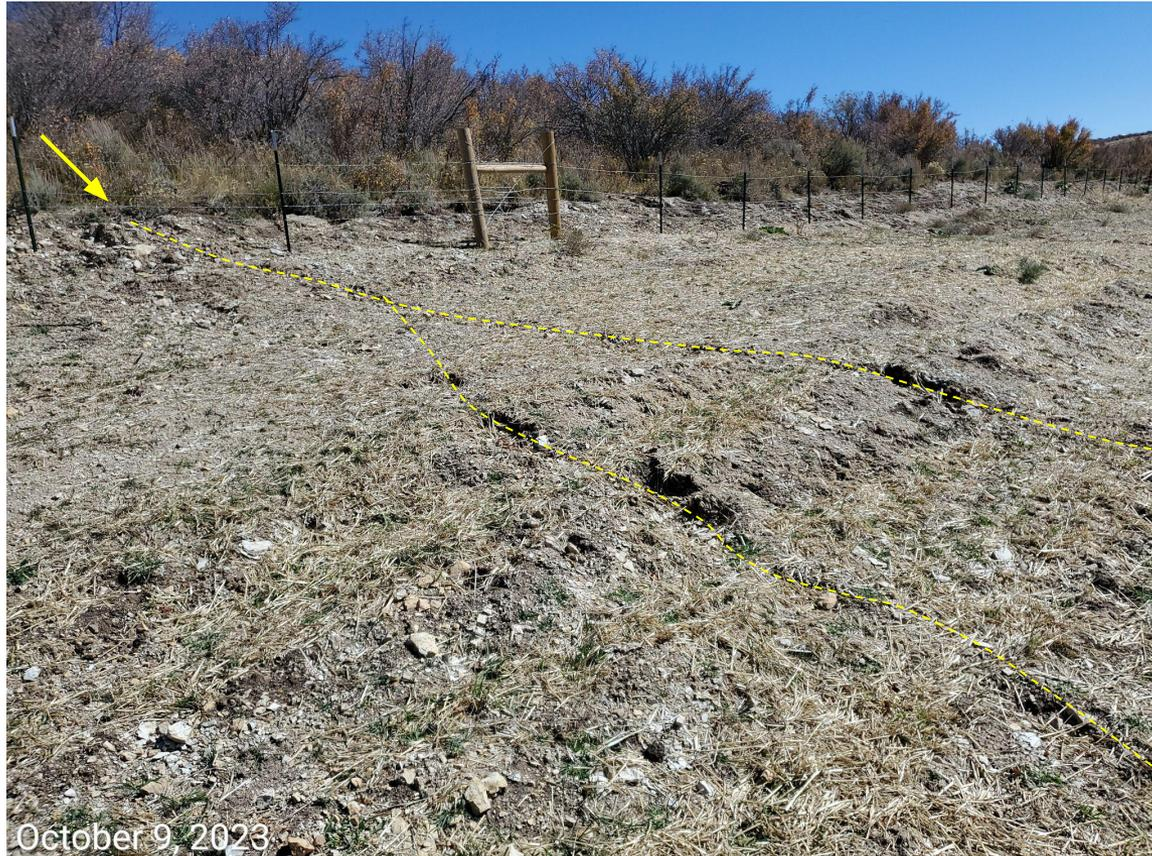
**Photo 10:** Photo example showing erosion degradation is becoming apparent. Perimeter control measures to manage runoff have not been implemented. Yellow arrows represent flow direction; lines outline erosion.
