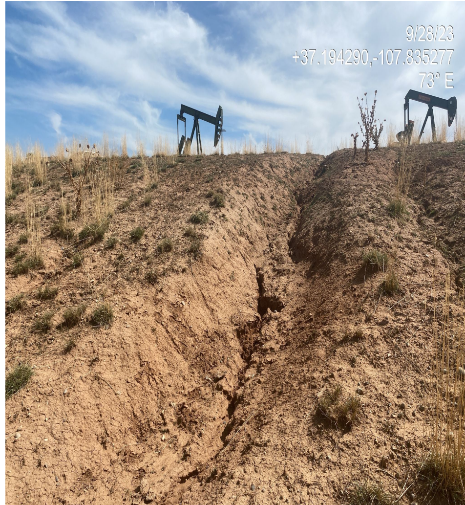
Photo 5. Photos of rill and gully erosion forming along western fill slope interim area.
