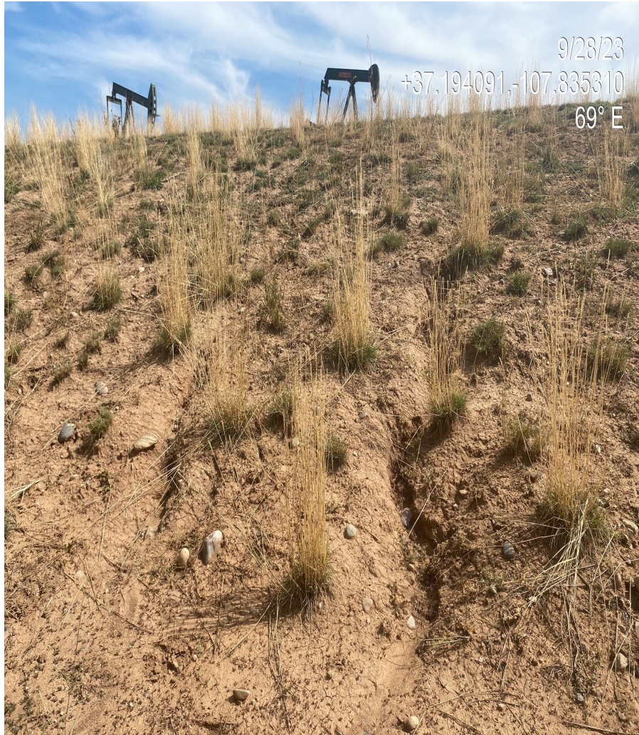
Photo 5. Photos of rill and gully erosion forming along western fill slope interim area.
