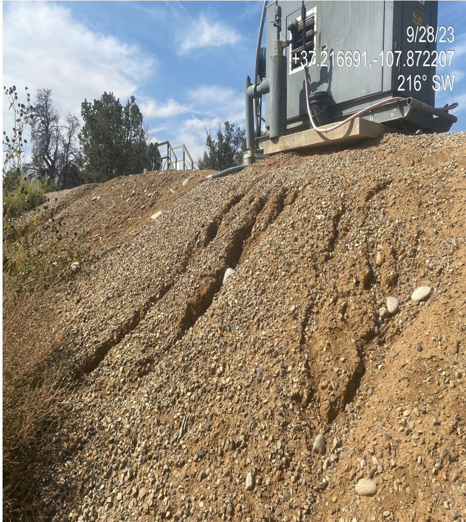
Photo 3. Rill erosion observed in several locations along the fill slope located on the eastern edge of the disturbance.
