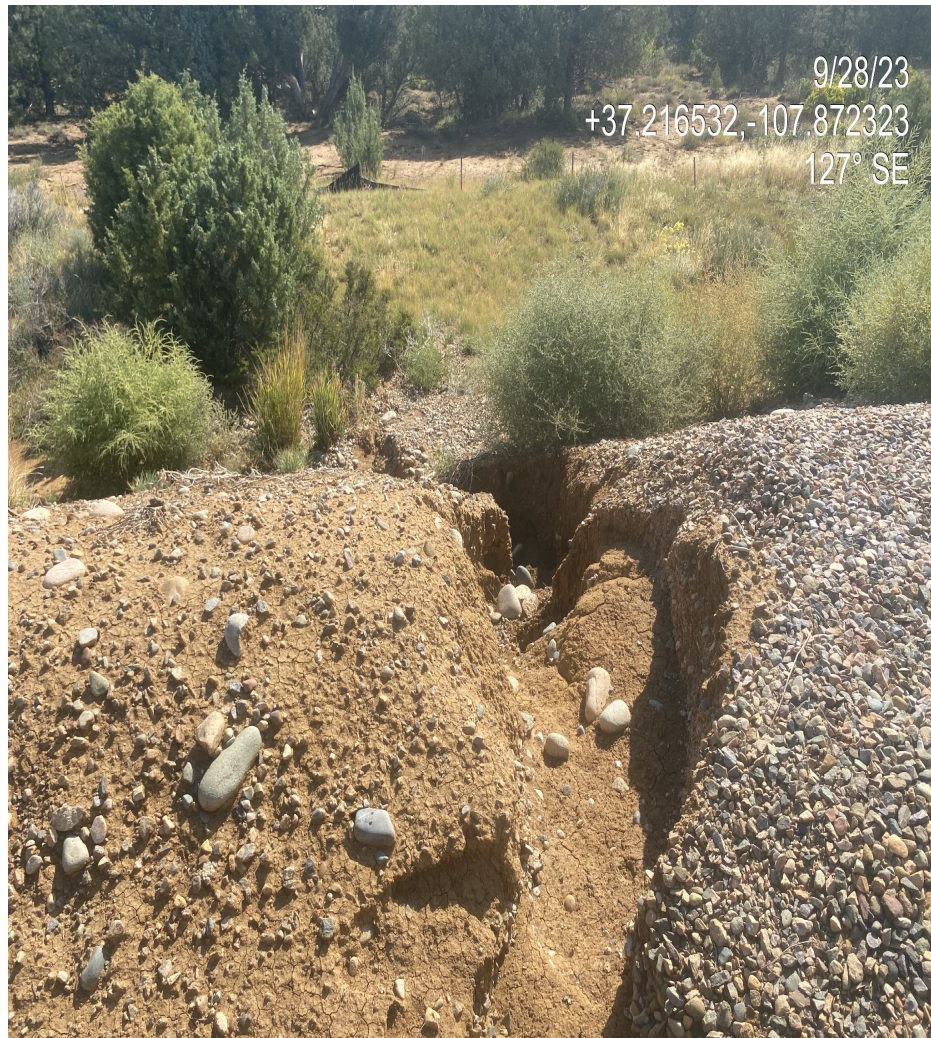
Photo 2. Photo of gully erosion observed on the fill slope, located on the eastern edge of the disturbance.
