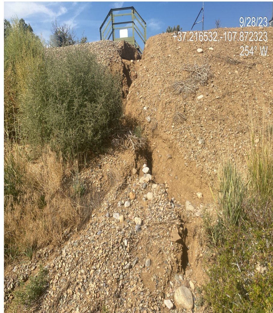
Photo 2. Photo of gully erosion observed on the fill slope, located on the eastern edge of the disturbance.
