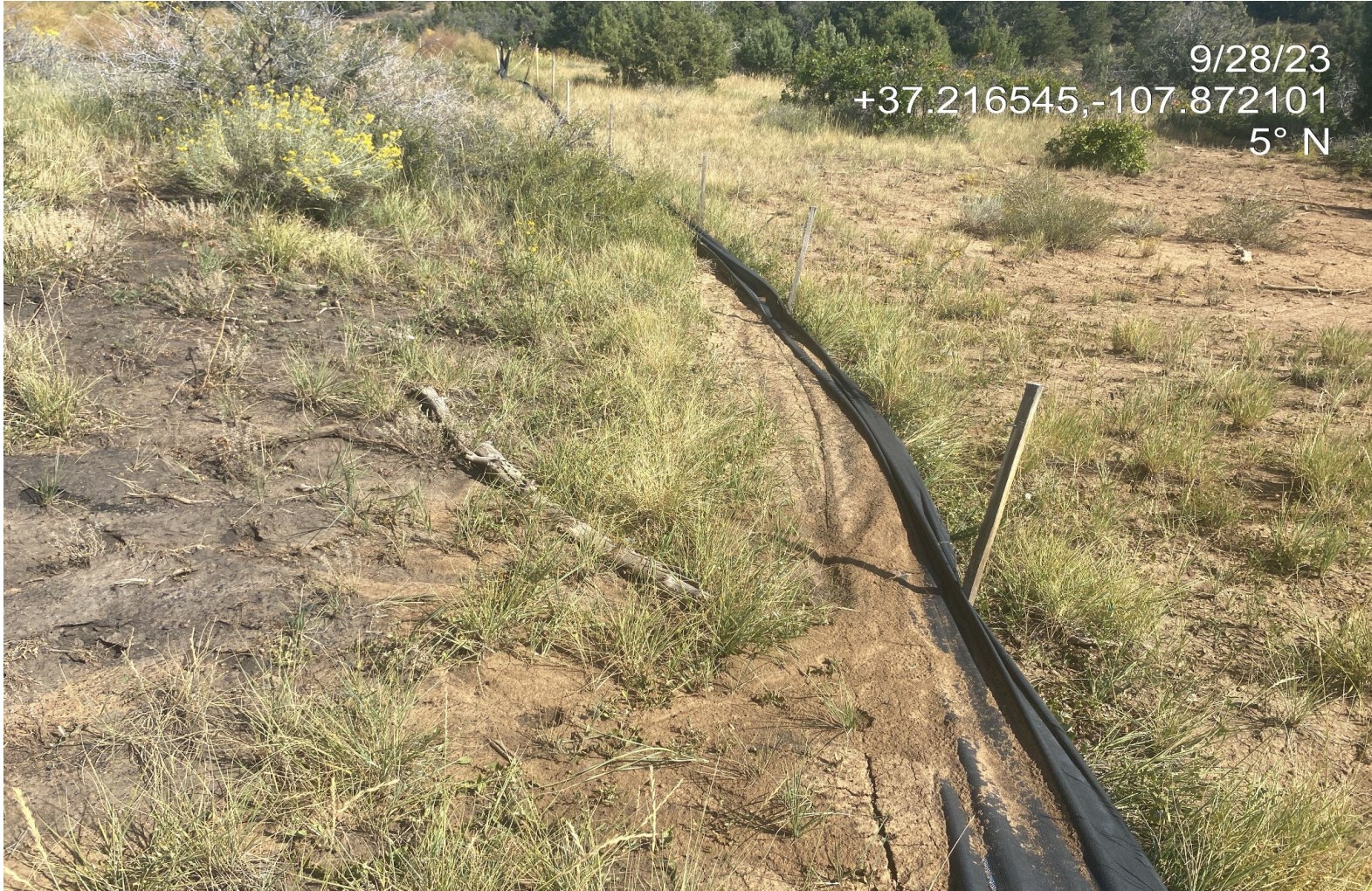
Photo 4. Silt fence along eastern edge of disturbance is in disrepair and is no longer functioning. BMP's used to minimize erosion and degradation of the location are inadequate.
