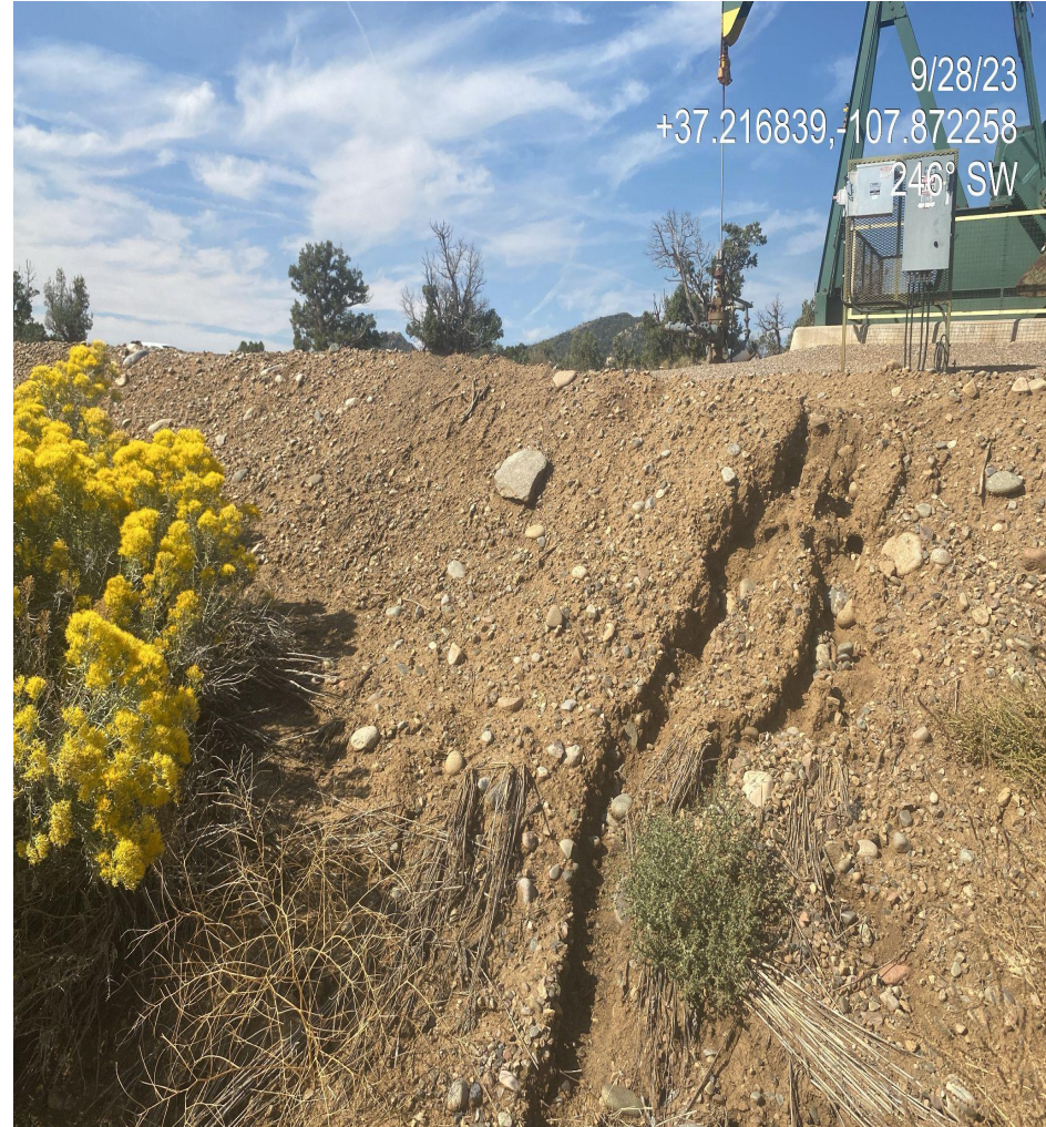
Photo 3. Rill erosion observed in several locations along the fill slope located on the eastern edge of the disturbance.
