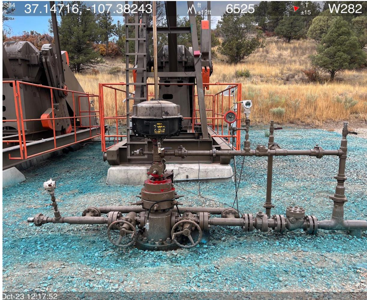
Photo #5 View of wellhead assembly.
