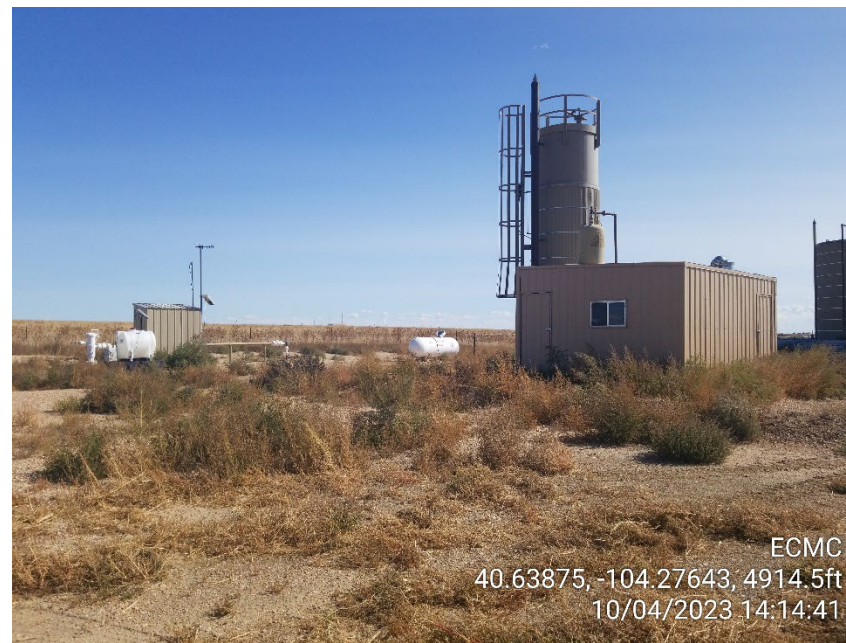
Photo 10 – Overgrown Vegetation at Heater Treater and Propane Tank
