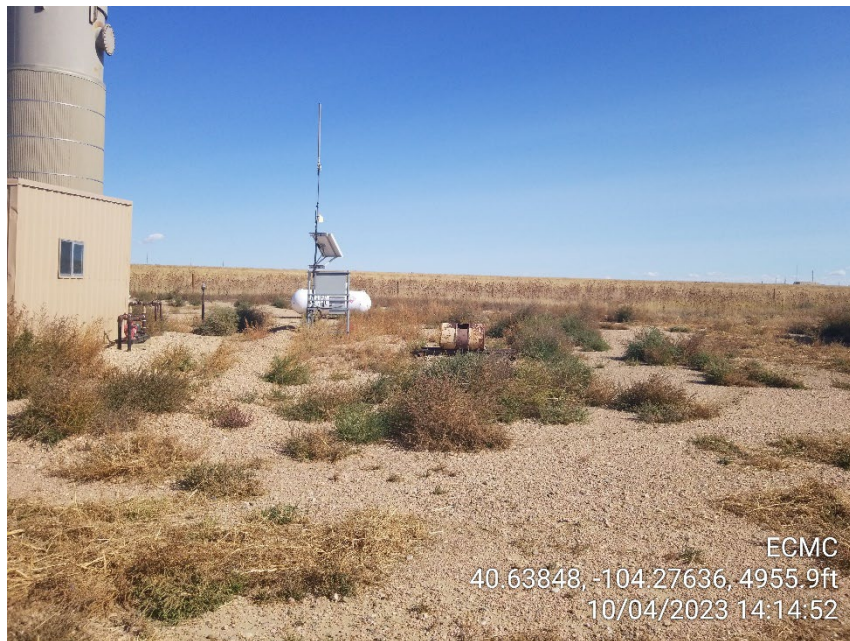
Photo 11 – Overgrown Vegetation at Heater Treater and Propane Tank
