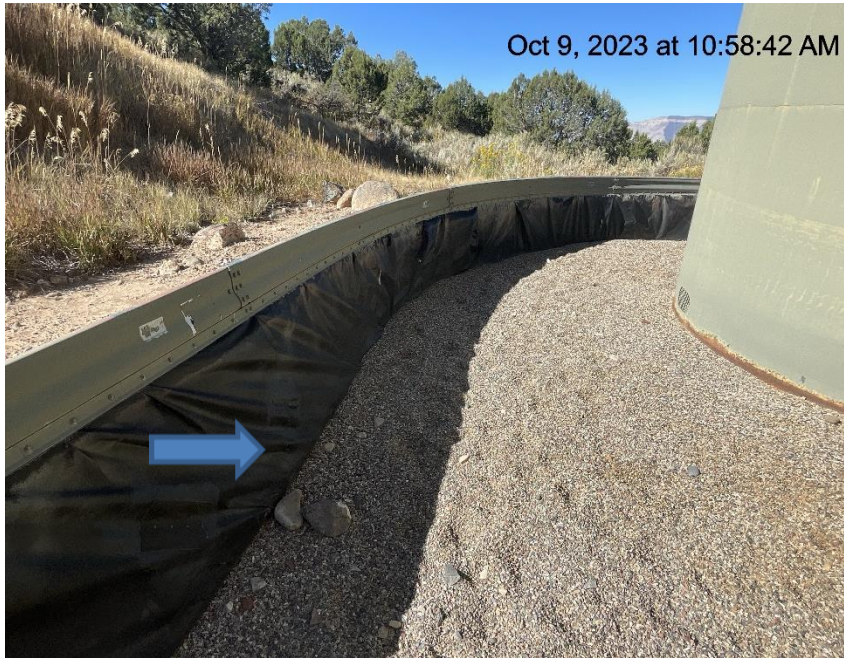
Photo # 1998 Hole in liner/liner needs maintenance
