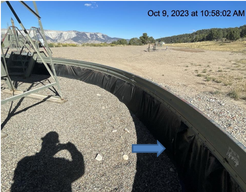
Photo # 1996 Hole in liner/liner needs maintenance
