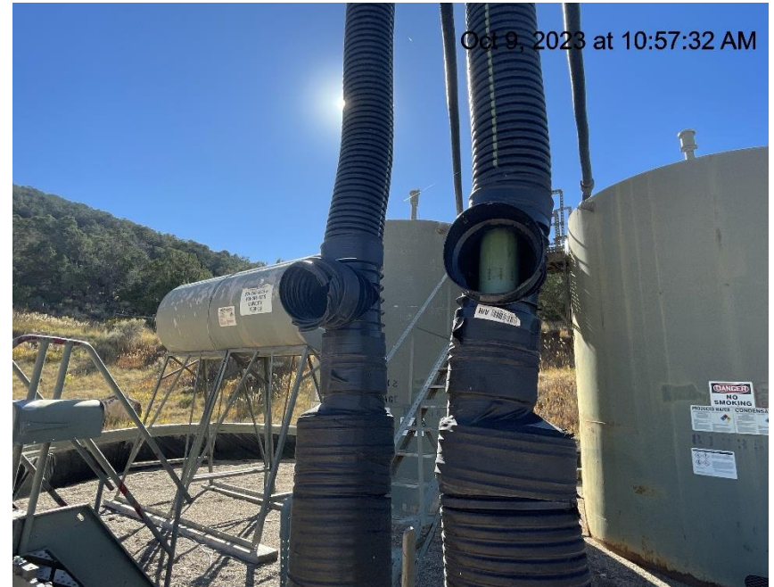
Photo # 1995 Flowline heating insulation open ended
