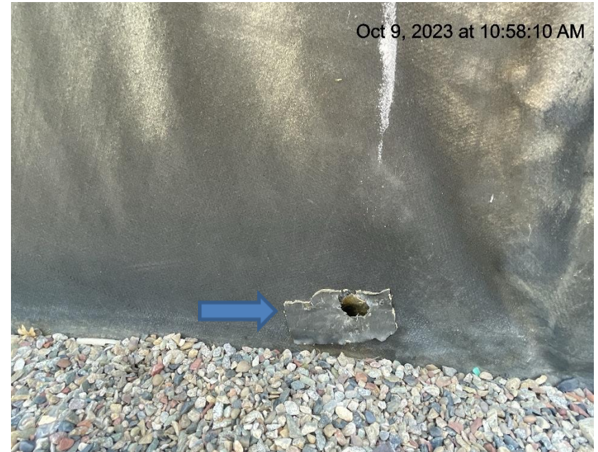
Photo # 1997 Hole in liner/liner needs maintenance
