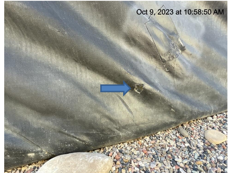
Photo # 1999 Hole in liner/liner needs maintenance
