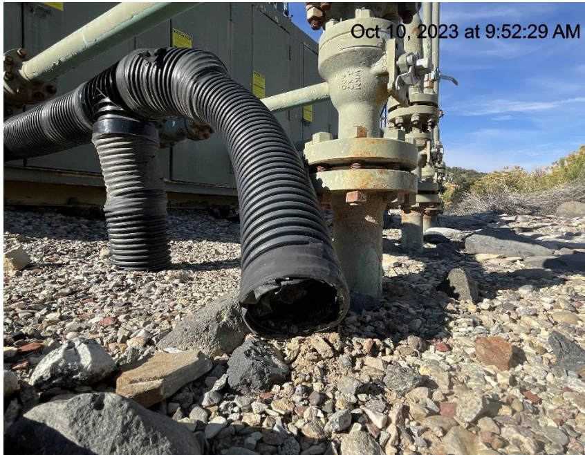
Photo # 2152 Flowline heating insulation open ended
