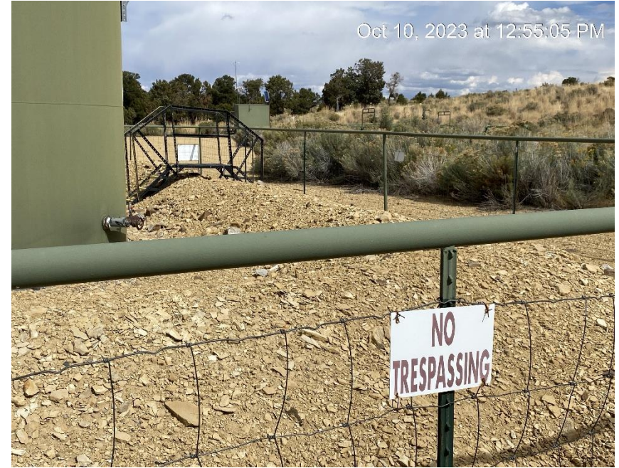
Location from Northwest corner
