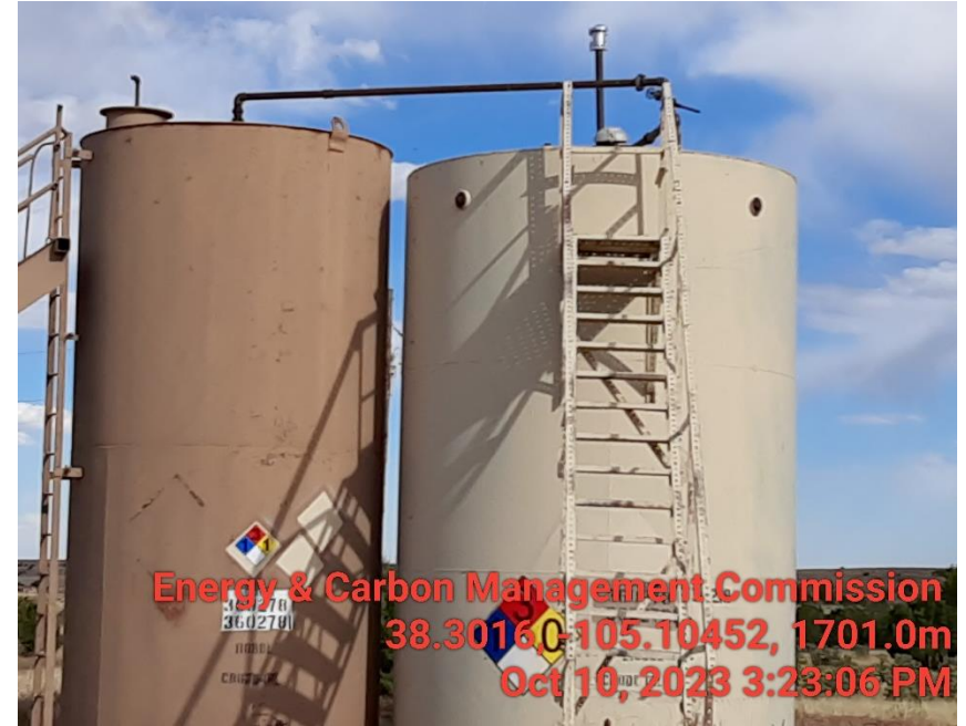
Photo 2 new NFPA placards and PRV installed
