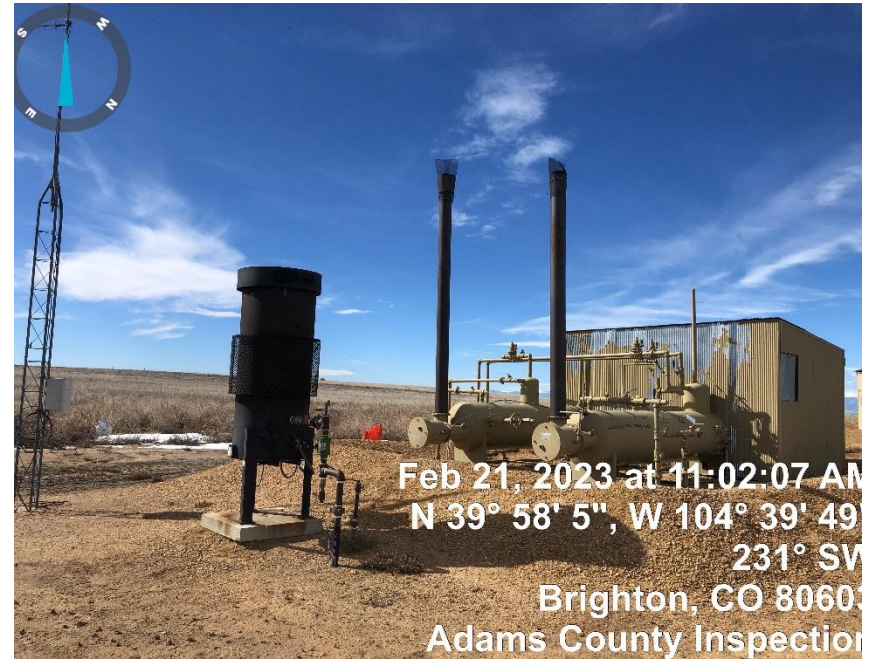
Photo#2 ECD/Separators/Automation Tower
