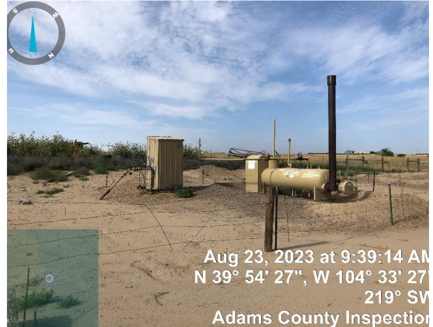
Photo#2 Gas Meter/Separator
